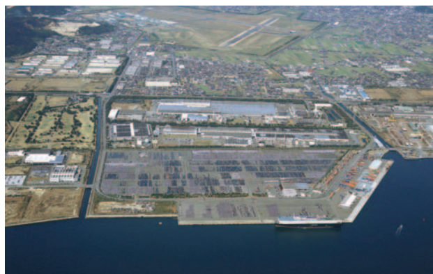
Hofu Plant, Nakanoseki District
