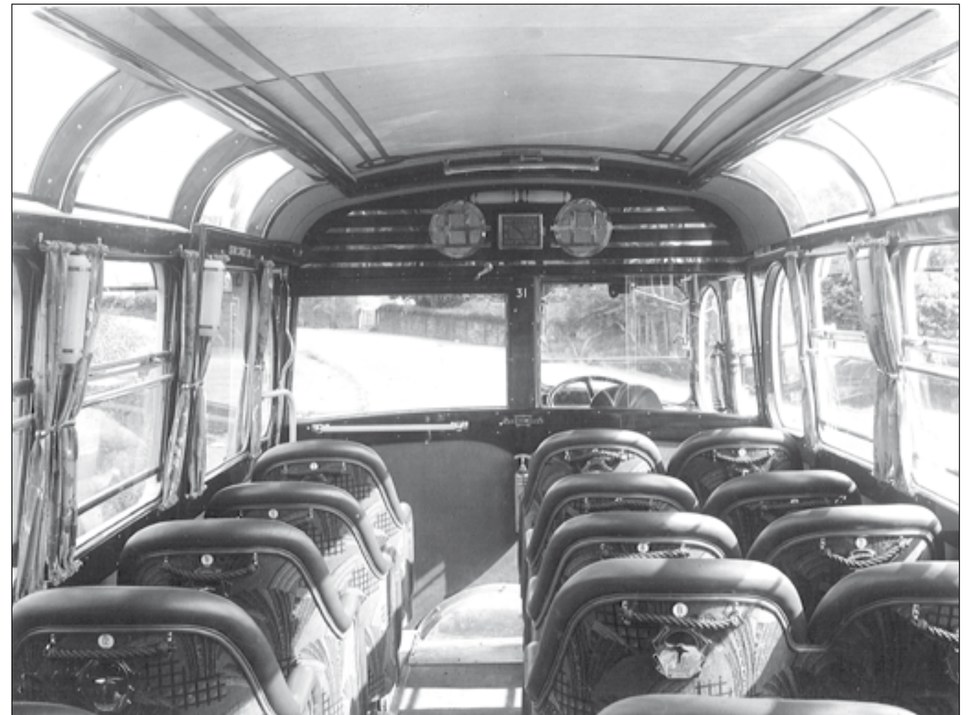
Cumberland No. 31 may have needed a Cov-Rad radiator conversion, and spats to cover the projecting dumb irons of its 1929 built chassis, but no one could fault the interior body appointments. Two-and-one deep leather-trimmed moquette seats with arm rests, radio speakers and a clock, glass cantrails for better visibility in the glorious Lake District, curtains to the deep half-drop windows and a discrete measure of chromium trim put this in a top quality league. Note the Massey Bros. gilt transfer on the bulkhead above the chrome fire extinguisher.
