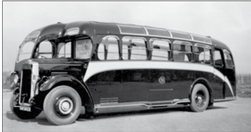
Seen at Keswick Bus Station about to depart for Borrowdale and Seatoller was Cumberland Motor Services No. 30, a Leyland TS2 dating from 1929. Its original Massey bus body was replaced by this Massey dual-purpose version in 1939 and it remained in service until 1949. The official view of No. 94, (RM 5629), left, shows more clearly the glass cantrail lights and glass louvres over the windows and the sloping roof line, whilst the familiar D-shaped windows are also prominent. Note that a neat entwined logo has replaced the former large bold CUMBERLAND lettering on the side panels – clearly this was felt to be more appropriate to a vehicle acting as a coach – even if only in disguise. The deep Cov-Rad radiator conversion was an attempt to modernise the frontal appearance of the long-outdated chassis.
