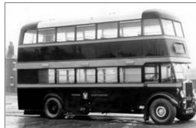
Widnes Corporation bought their first of many Leyland double-deckers in November 1936. This is No. 42, BTD 123, and it was one of five Leyland Titan TD4 type with highbridge 52-seat bodies, again seen at Enfield Street prior to delivery.
