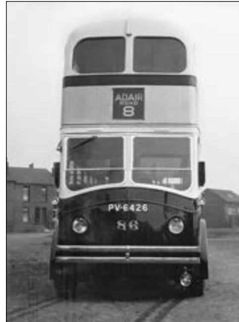
Ipswich No. 86 bodied by Masseys in 1940 was a Ransomes, Sims and Jefferies trolleybus built as a demonstrator for a tour of South Africa, but due to the outbreak of World War Two was diverted by the MoWT to Ipswich Corporation. It was the last Ransomes vehicle to enter service with a British operator, was the last trolleybus to be bodied by Massey Bros, and was withdrawn and scrapped in September 1959.
