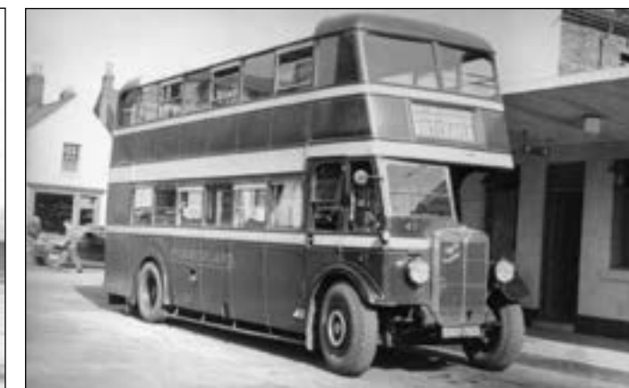
Cumberland's AEC Regent demonstrator, number 47, was replaced by another AEC Regent when it was sold in 1936. Also numbered 47 and also bodied by Massey BAO 763 was one of a pair, 12 and 47, with the current lowbridge body design as shown here. (JFH)
