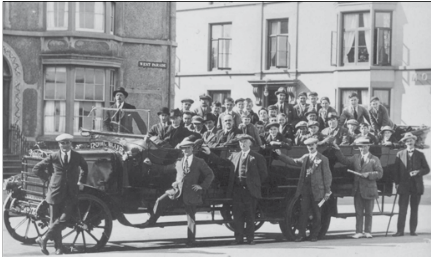
This Daimler B-type started life in London before being purchased by Royal Blue in Llandudno, North Wales, and fitted with a charabanc body as seen here in Rhyl. The robust, if somewhat rudimentary, chassis, was capable of more than seasonal summer excursion work, of course, and like many others purchased in the early post-war years was soon rebuilt as a saloon bus. This example was rebodied with a Massey 32-seat body as seen below in May 1922 for new owners Brookes Brothers based in Rhyl. Trading as White Rose Motors the firm grew to an impressive size and became a considerable thorn in the side of the Crosville Motor Company until the takeover after the LMSR investment in Crosville. The company had considerable charisma and one of its mid-twenties Leyland-bodied Leyland SG-types has been lovingly restored by Mike Sutcliffe, the Leyland specialist, ensuring this splendid livery and much-loved operator will not be forgotten. (STA upper)
