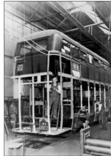
When a professional photographer was brought into the body shop at Enfield Street to record this scene it could only have been a sign that something was afoot; the cause celebre in this instance was Bolton Corporation No. 119, a Leyland Titan TD5c delivered to the operator in September 1937, and seen here being completely reframed in the lower-deck. In today's compensation culture climate this might be evidence for a claim against the timber supplier – was it indeed just that we wonder?
