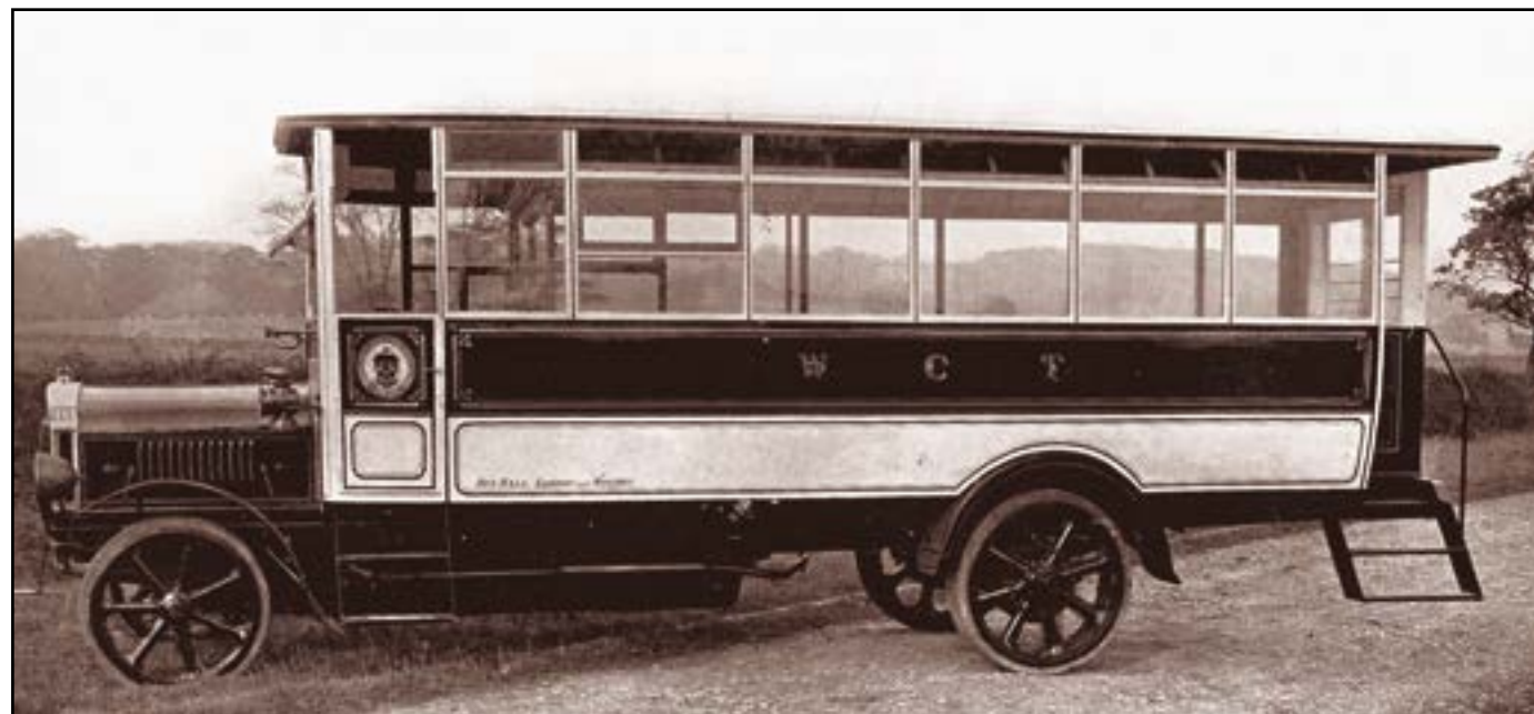
Wigan Corporation's Tilling-Stevens petrol-electric chassis were fitted with dual-doorway bodies as seen here, but had short lives as noted in the text. The half-open rear was quite common at the time, being favoured by several bodybuilders. Note the high floor, requiring steps for access, due to the straight-framed chassis – a normal feature until cranked chassis were introduced later in the 1920s.
