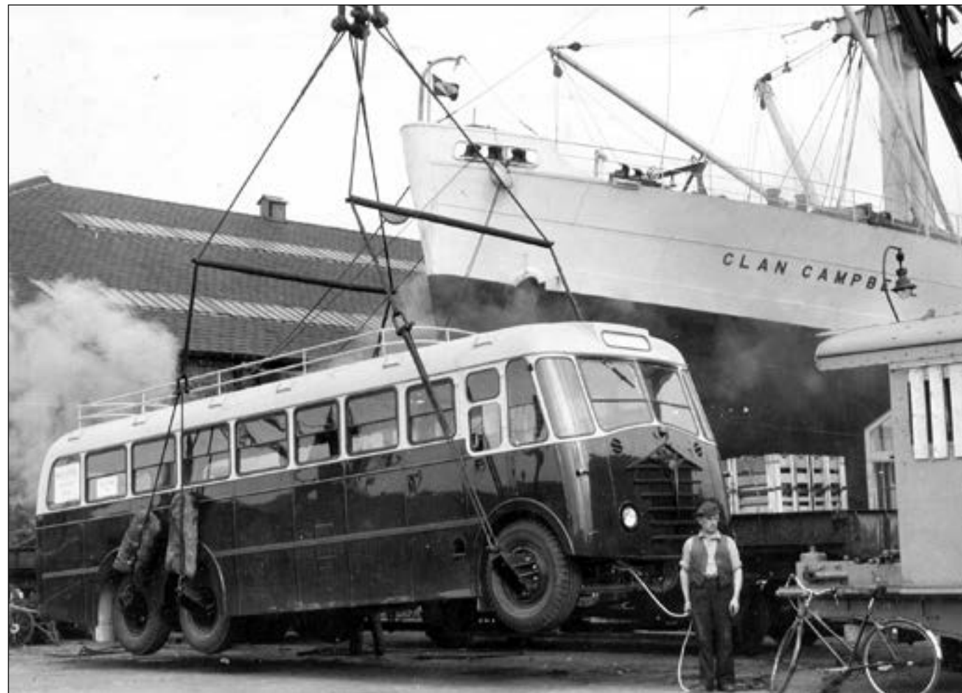
In 1954 Massey Bros. received an order for the building of eight 53-seat bus bodies on specially adapted Foden FG6/12 commercial chassis for the Lourenco Marques section of the Mozambique Railways. Two are seen in build, above, whilst a completed example is shown below about to be hoisted aboard the ship before its long sea voyage on one of Clan Lines' vessels.
