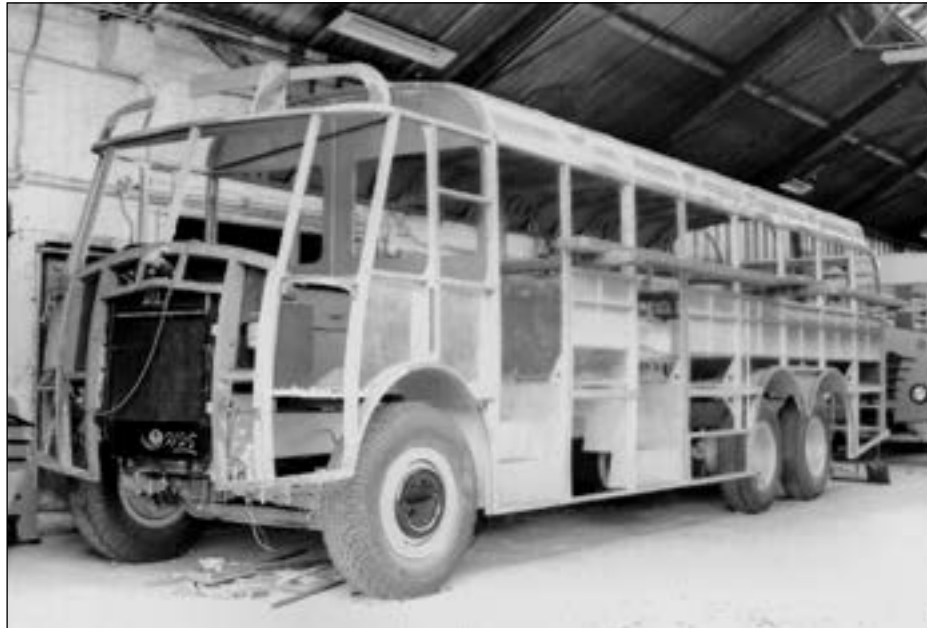
In 1954 Massey Bros. received an order for the building of eight 53-seat bus bodies on specially adapted Foden FG6/12 commercial chassis for the Lourenco Marques section of the Mozambique Railways. Two are seen in build, above, whilst a completed example is shown below about to be hoisted aboard the ship before its long sea voyage on one of Clan Lines' vessels.
