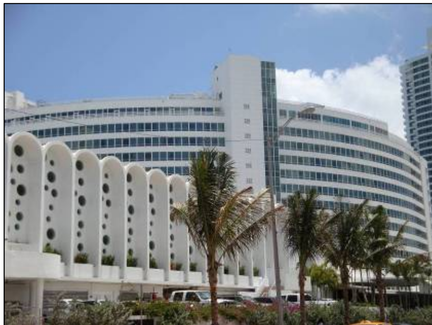
Fontainebleau Hotel. Morris Lapidus designed Chateau (1954) and A. Herbert Mathes designed North addition (1959), located at 4441 Collins Avenue
