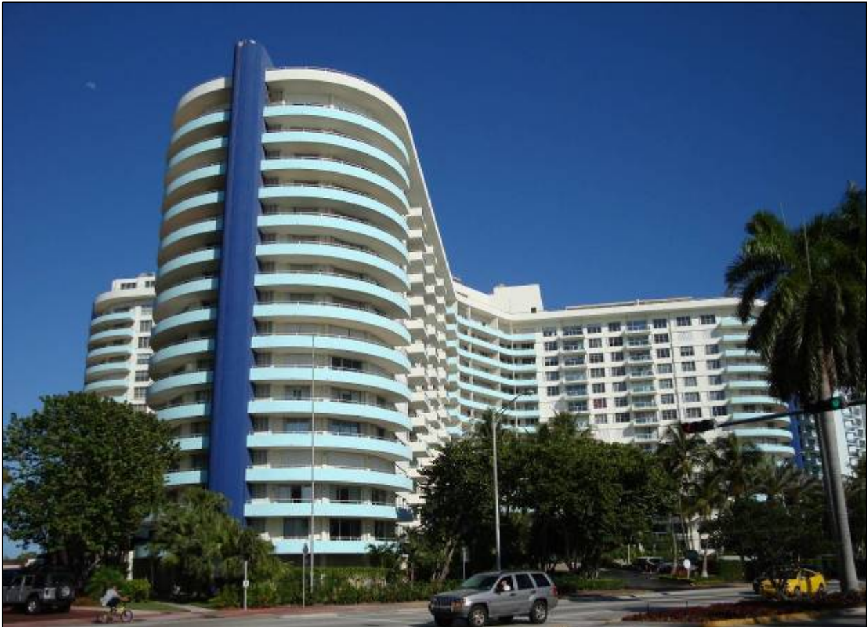
Seacoast Towers East designed by Morris Lapidus in 1965 located at 5151-5161 Collins Avenue
