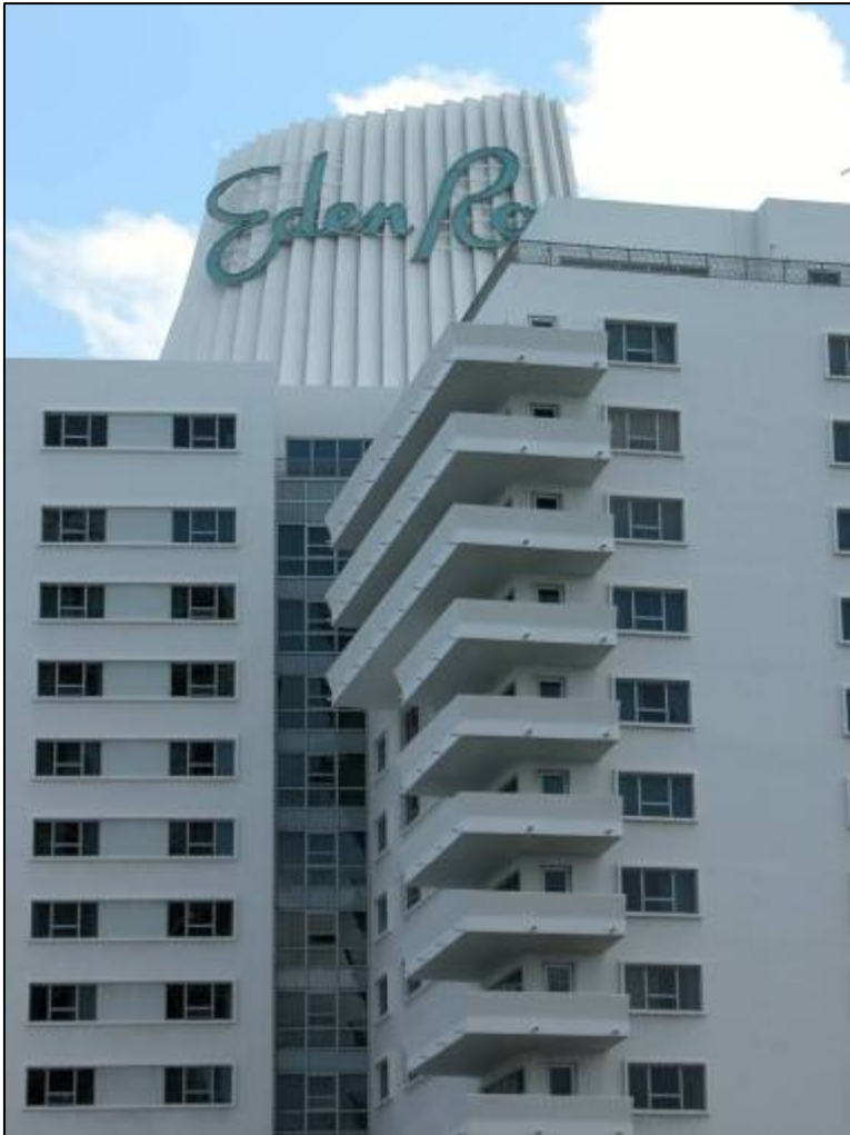
Eden Roc Hotel with cantilevered balconies, ships roof-top funnel, mosaic tiles and molded concrete tracery.
