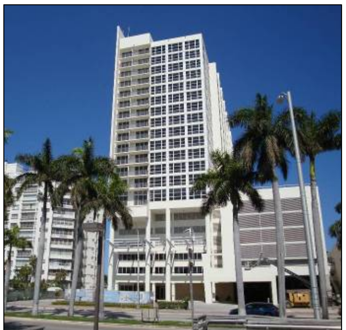
Grand Beach Hotel, under construction 4835 Collins Avenue
