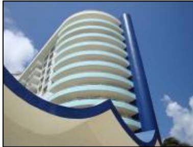
Seacoast Towers East, designed by Morris Lapidus
