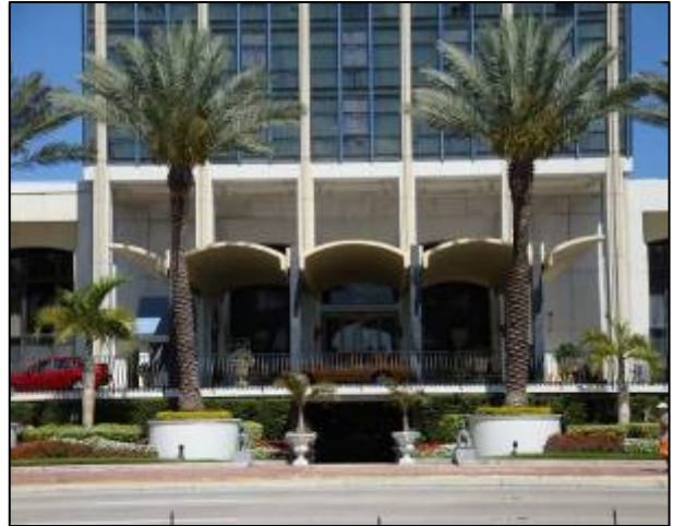
Doral Beach Hotel entry with a cantilevered canopy of continuous arches.
