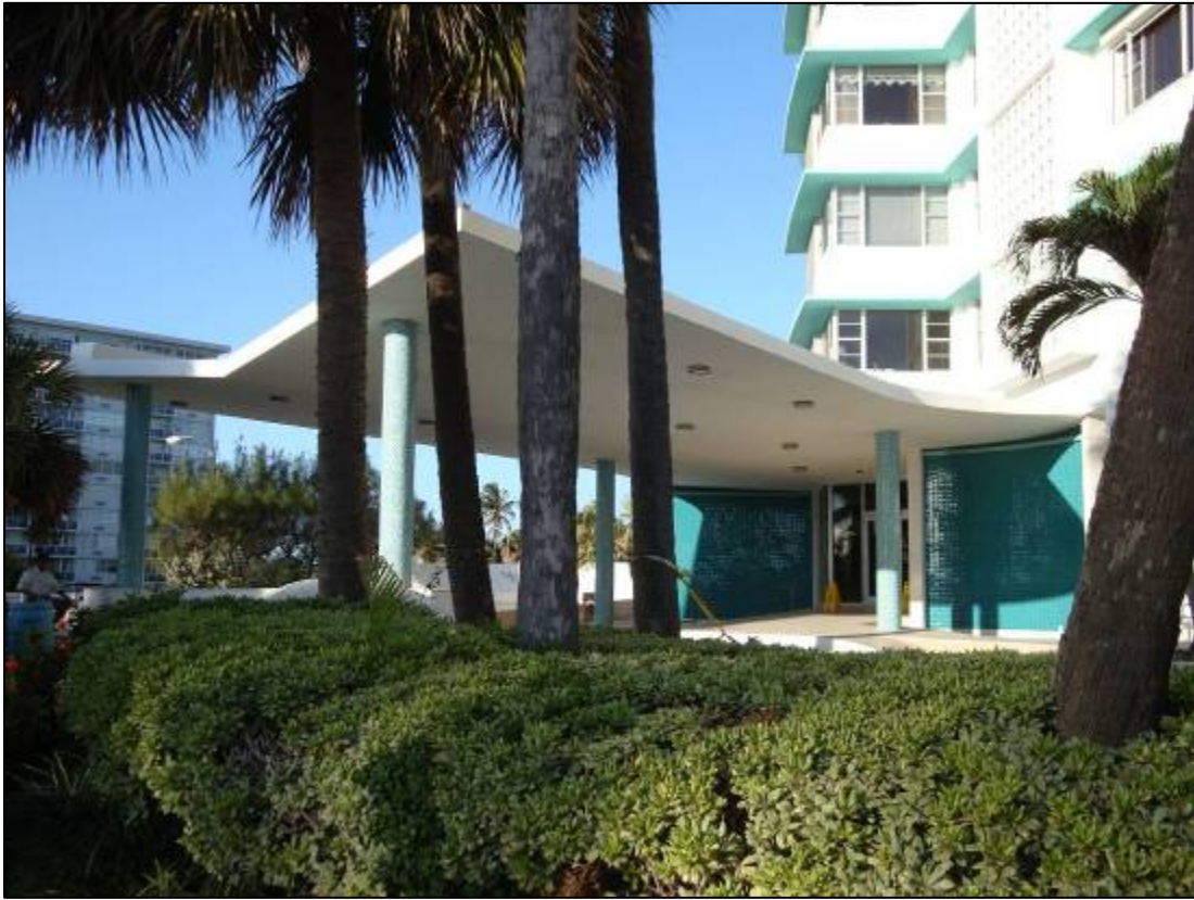
Dramatic entry porte-cochere at Imperial House, reconstructed 2009.
