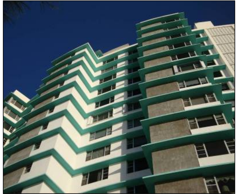
Curved front façade of the Imperial House with continuous masonry eyebrows.
