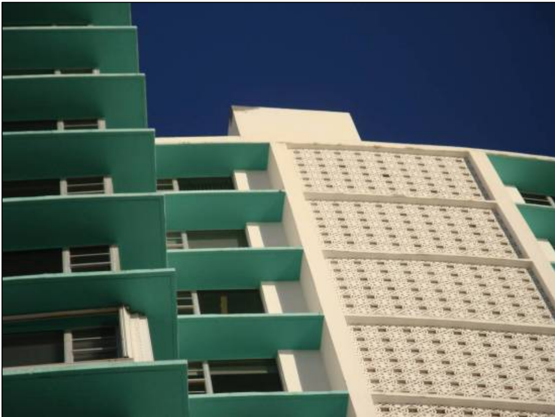
Imperial House, detail of breeze-block and 'eyebrows'
