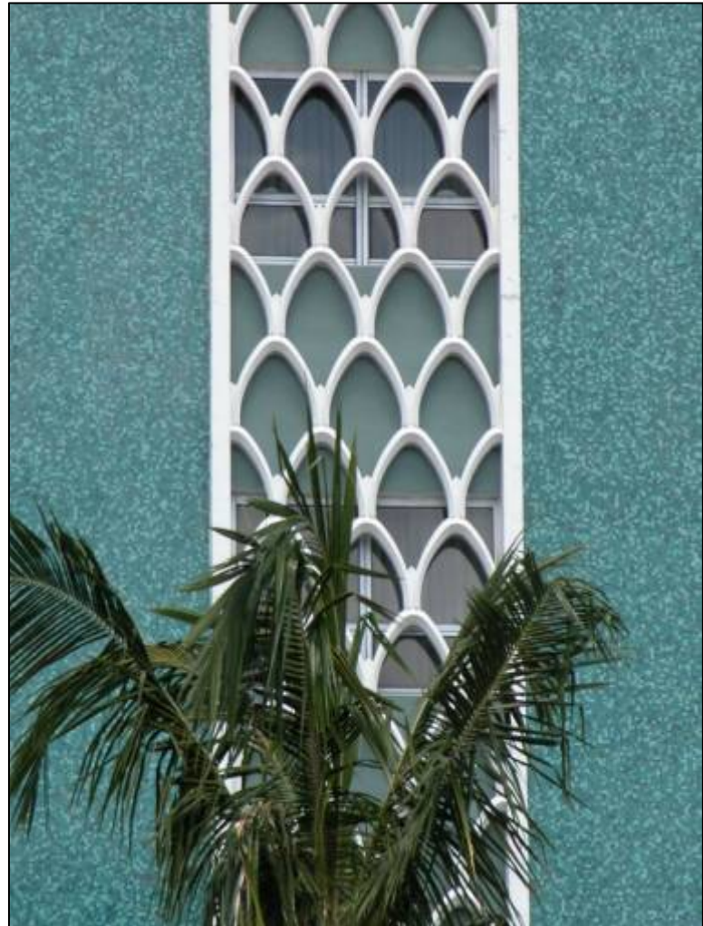
Eden Roc Hotel with cantilevered balconies, ships roof-top funnel, mosaic tiles and molded concrete tracery.
