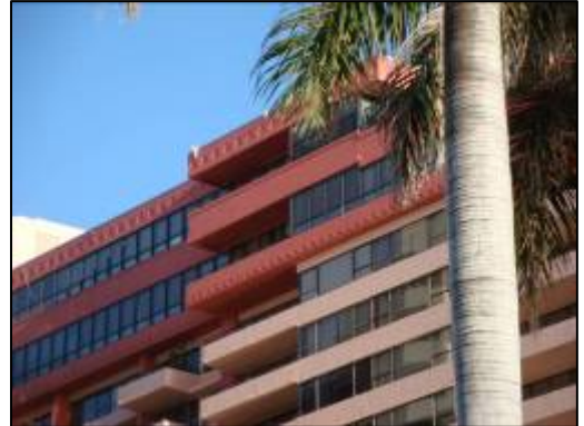
The Alexander, balcony detail
