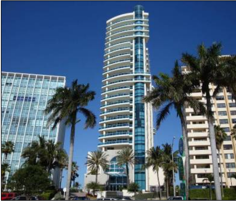
Capobella, constructed 1992 5025 Collins Avenue
