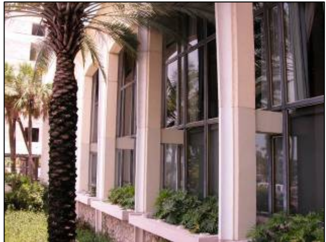
Doral Beach Hotel with its slender piers of precast quartz stone
