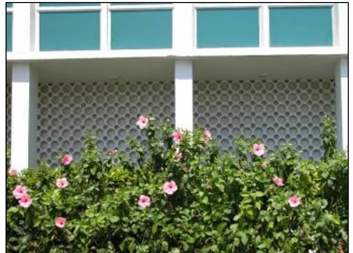
Crystal House, panels of perforated masonry in a pattern of regimented cheese-holes, fronting Collins Avenue.
