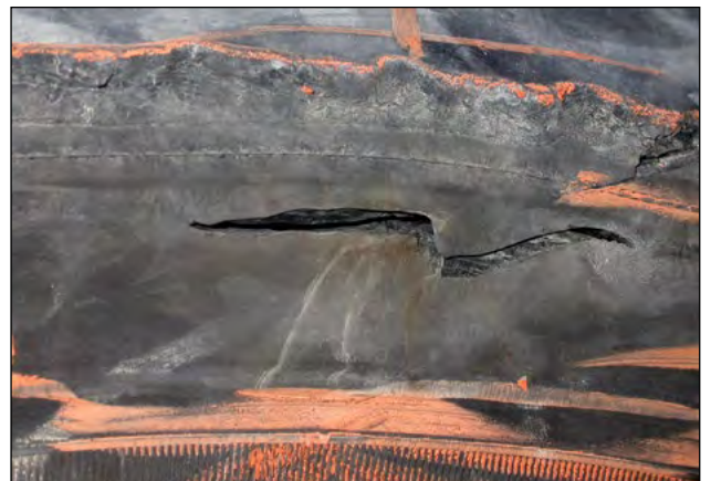
Sidewall Damage from Impact
