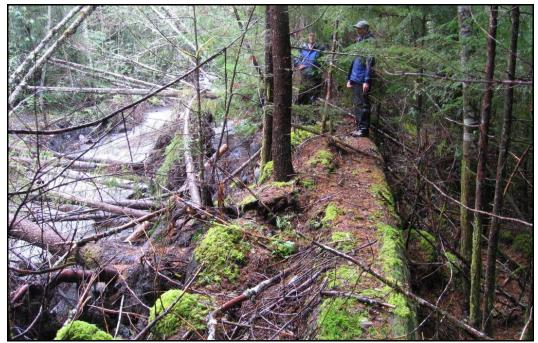
Figure 21. FS2008-10 Log and Boulder Levee. Burtchard and Gleason stand on cabled logs.
