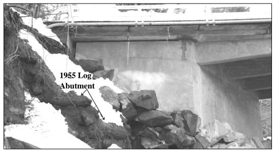
Figure 24. 1955 Kautz Creek Log Bridge Abutment Adjacent to the 1964 Concrete Bridge
