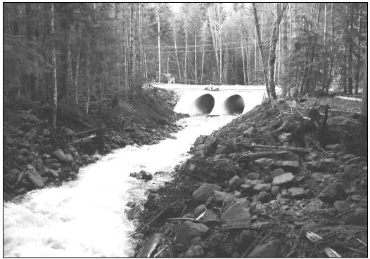
**Figure 25.** New Kautz Creek and Culverts in May 2007. Log-backed levee site FS2008-10 is located on the right (east) side of the creek, approximately 200 feet upstream (north) of the road.
