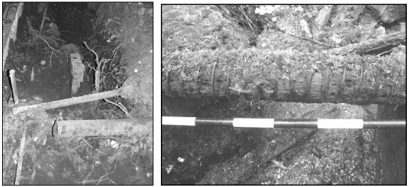
Figure 9. Wood-stave Pipe at Oscar Brown Cabin (lower left) and Crossing a Small Stream at Site FS2008-03 (Feature 2, right, scale in 10 cm increments)
