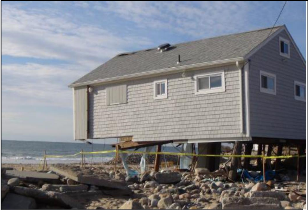
Figure 1-10: Damaged home in Westerly, Rhode Island after Hurricane Sandy (October 2012).
