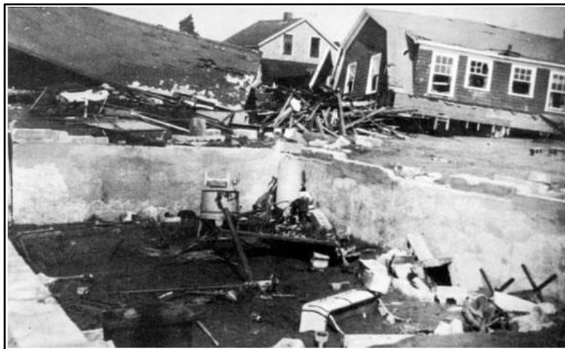
Figure 1-8: The remains of houses in Island Park, Rhode Island after the hurricane of 1938. (Source NOAA)
