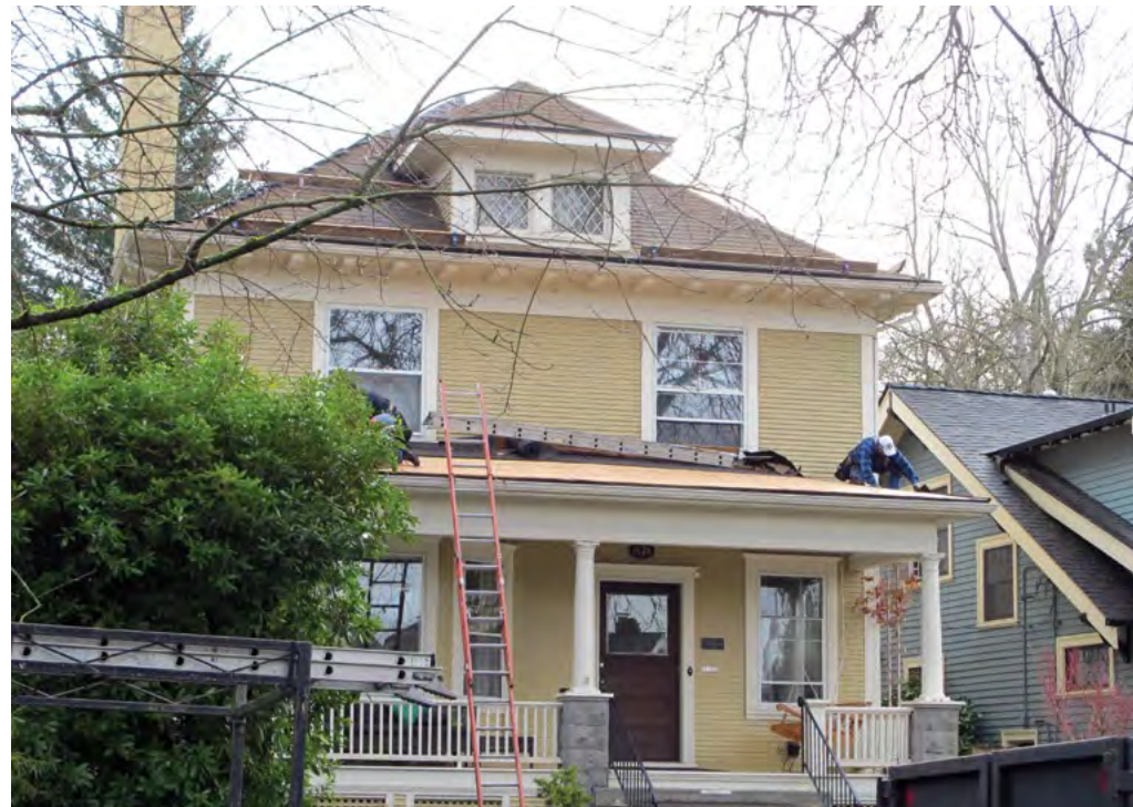
[16] The deteriorated asphalt shingles of this porch roof are being replaced in kind with matching shingles.
