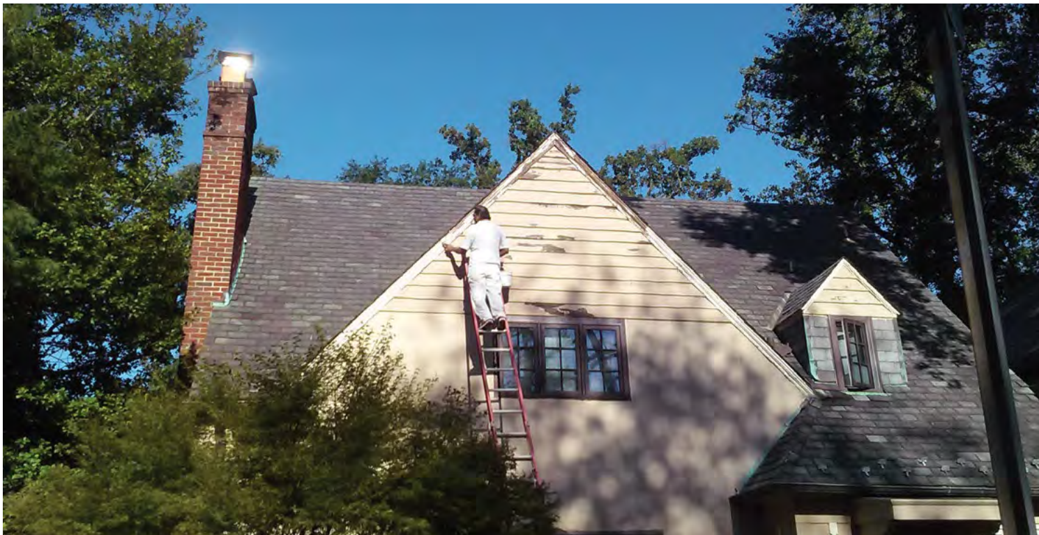
[4] Hand scraping to remove peeling paint from wood siding in preparation for repainting is an important part of regularly-scheduled maintenance.
