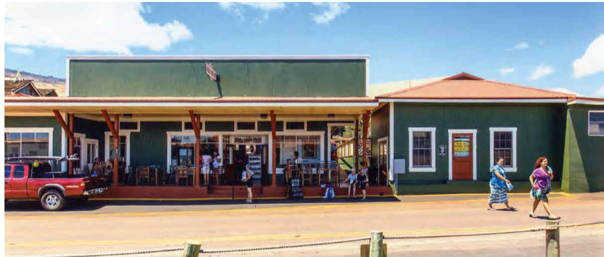
[29] The rehabilitation of the 1910 Māālaea General Store (a), which served the workers' camp at the Wailuku Sugar Company on the Hawaiian island of Maui, included the reconstruction of the original parapet (b).
