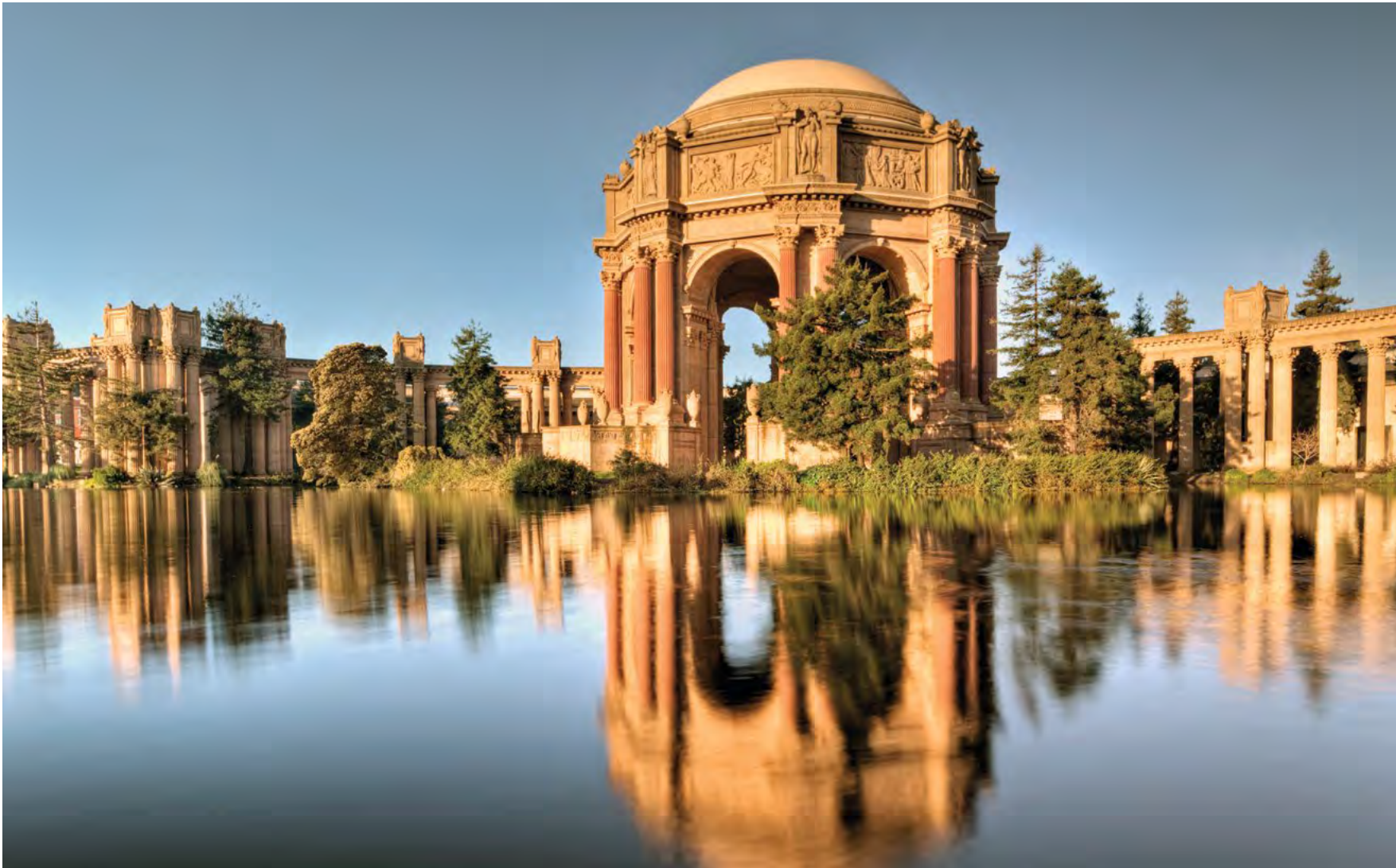
[8] The Palace of Fine Arts was designed by Bernard Maybeck and built for the 1915 Panama-Pacific Exposition in San Francisco. The pavilion was intended to be temporary and, although it had a steel structure, the exterior was finished only with stucco, an impermanent material composed of plaster and fiber. The building was not torn down after the exposition, and it eventually fell into ruin. In 1964, all but the steel structure was demolished, and the building was reconstructed with lightweight poured-in-place concrete. Photo: KevinCole at Wikimedia Commons.
