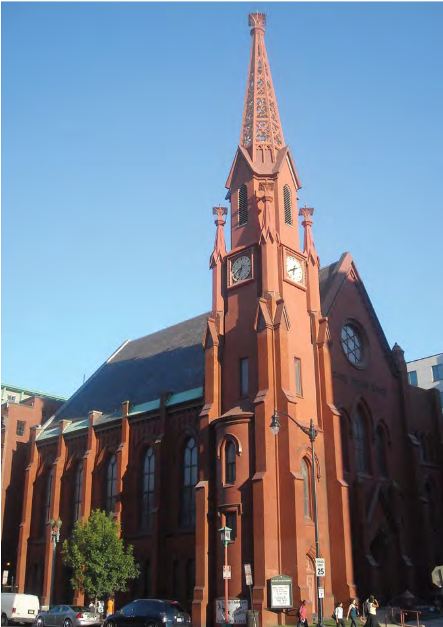
[8] The missing steeple of this historic church was replaced with a new steeple made of a substitute material that, from the street below, closely resembles the original steeple. Photo: en.Wikipedia.
