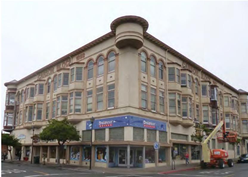
[32] (a-b) The rehabilitation of the 1892 Carson Block Building in Eureka, CA, for its owner, the Northern California Indian Development Council, included recreating the missing corner turret and sensitively introducing seismic reinforcement (c) shown here (opposite page) in a secondary upper floor office space. Photos: Page & Turnbull.
