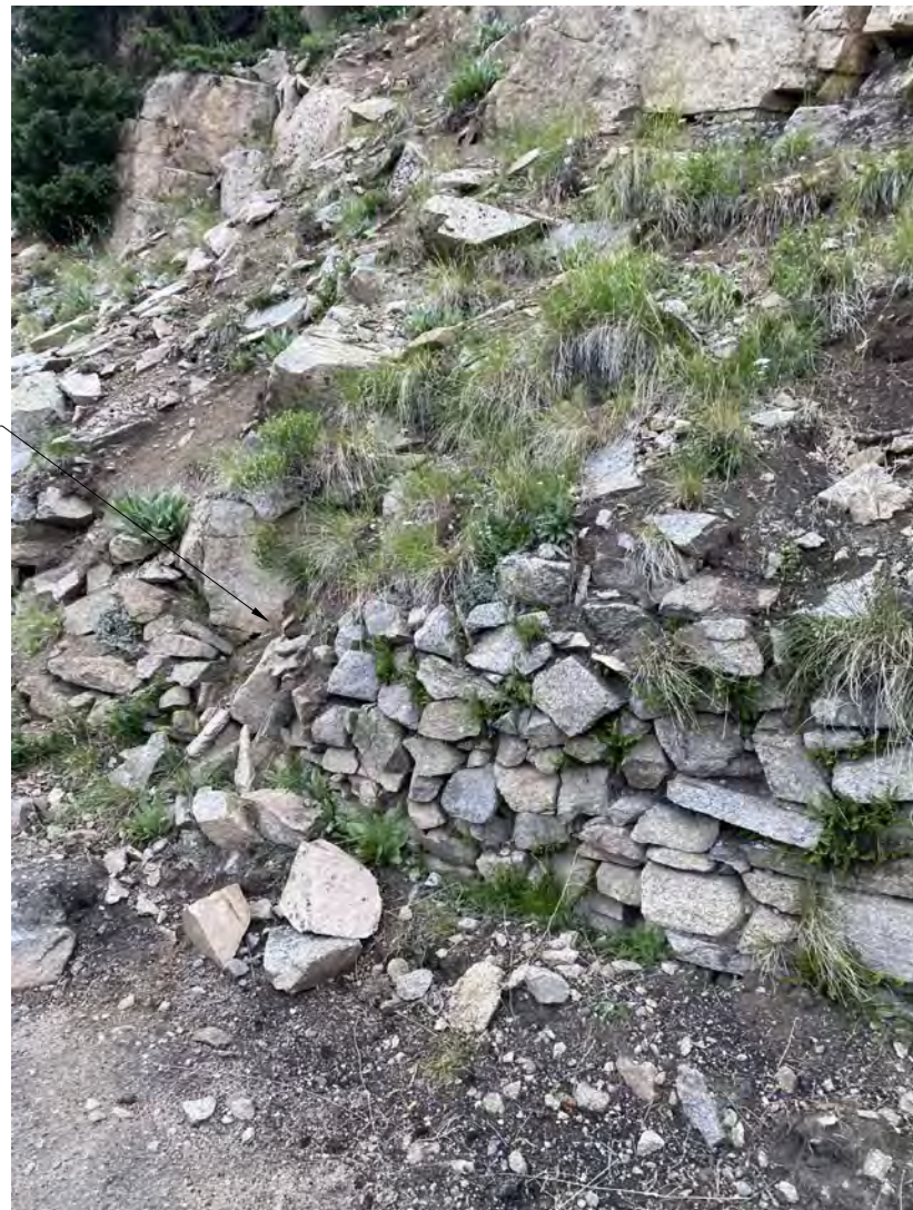
2 OPTIONAL BID ITEM - BREAST WALL REPAIR NEAR COLLAPSE PHOTO NO SCALE
