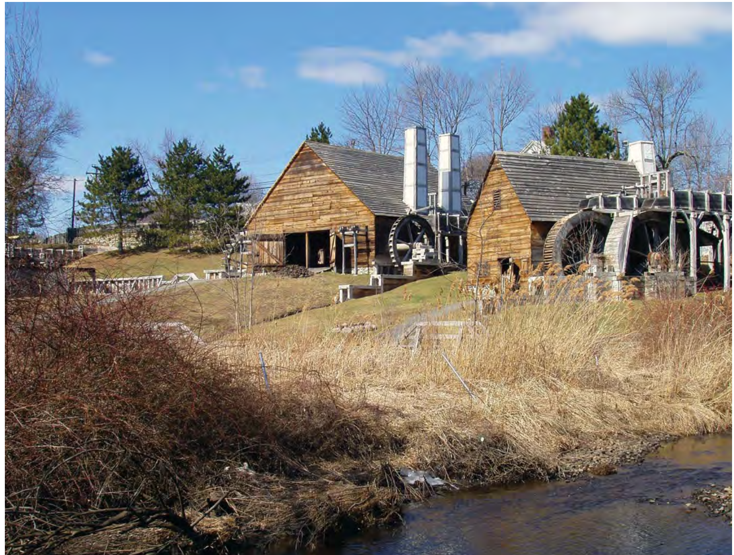
[2] The Saugus Iron Works, Saugus, MA, a National Historic Site, was active from 1646 to about 1670 and was the first integrated iron works in North America. The forge and mill (shown here) are part of the site which was reconstructed based on archeological research and historic documents and opened in 1954. Photo: Daderot at the English language Wikipedia.
