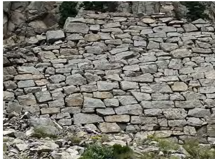
3 STONE COURSING EXAMPLE 1 PHOTO BELOW COLLAPSE 1/4" = 1'-0"
