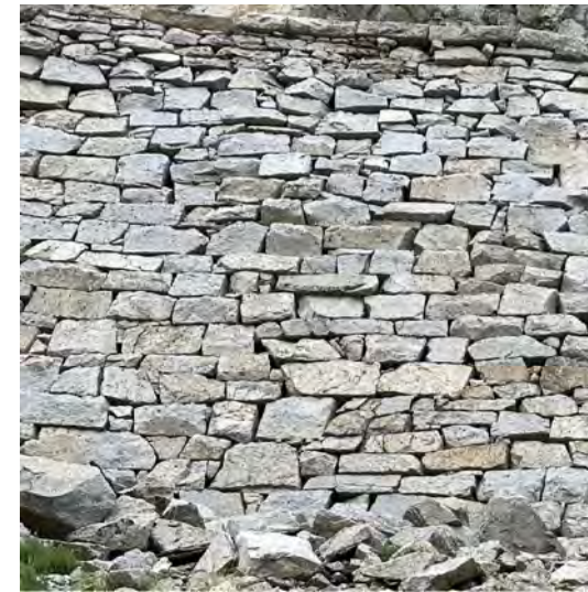
4 STONE COURSING EXAMPLE 2 PHOTO NEAR NORTH END 1/4" = 1'-0"
