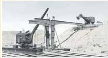
1939 East Ely Overpass
