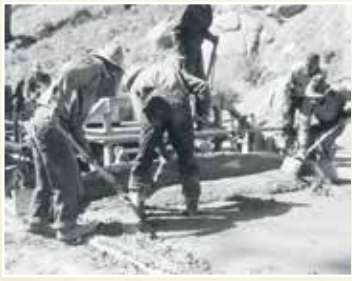
40s / 50s - Highway Paving Washoe County.
