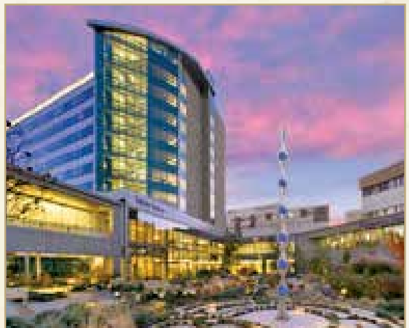
Renown Regional Medical Center Tower
