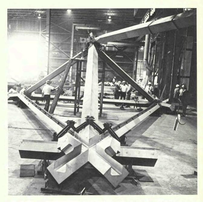
for the space frame of the East Building's huge skylight was inspected, procedures for erecting the space frame were reviewed, and the crane needed to install it began its journey to the site.
