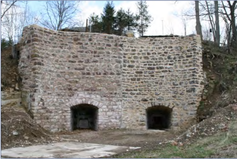
Somerset County's historic agricultural landscape is rich with many kinds of historic resources that evolved to support the farm industry. Such key elements as mills, lime kilns, forges, railroads, bridges, and even the Delaware and Raritan Canal enabled farmers to produce their goods and get them to market. Pictured here are the Moses Craig Lime Kilns, recently restored in Peapack (c. 1860); and Kline's Mill, a rare surviving early sawmill now serving as a residence, occupying a site known to host a water-powered mill since 1744. (Photos courtesy Somerset County Cultural & Heritage Commission)
