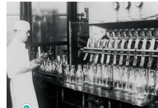
Bottling machines made milk easier to process and distribute, 1920s
