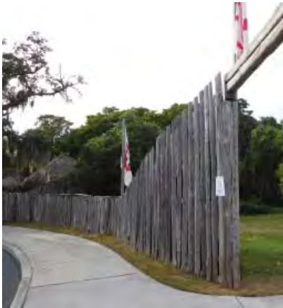
FIGURE 3-118. Palisade, view west-southwest at plaza entry.
