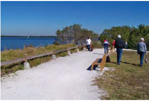
FIGURE 3-15. Top of berm (view east).
