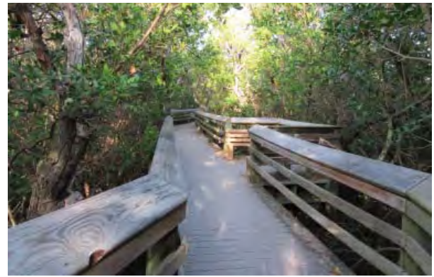
FIGURE 3-76. Boardwalk, view east, near midpoint.
