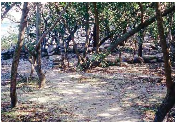
FIGURE 2-80. Staff formed these edging stones by filling sandbags with cement; here shown staged for use in reinforcing trail edges and a drainage channel, c. 2000-2005. (DESO Archives)
