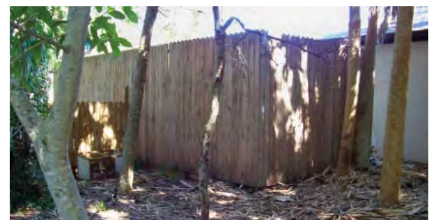
FIGURE 3-162. Wood privacy fence at west end of maintenance building, view northeast.
