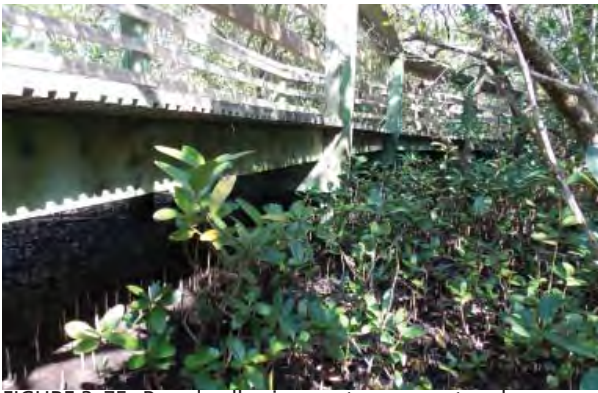
FIGURE 3-75. Boardwalk, view east, near west end.
