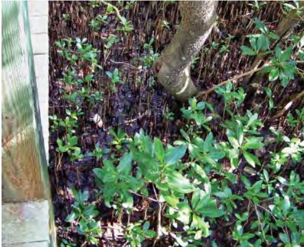
FIGURE 3-77. Adjacent ground, west end of boardwalk.
