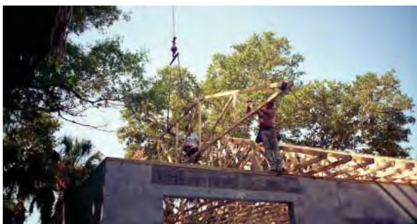
FIGURE 2-99. Maintenance building construction, 1994; view south. (DESO Archives)
