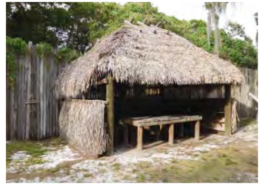
FIGURE 3-117. North chickee, view northeast.
