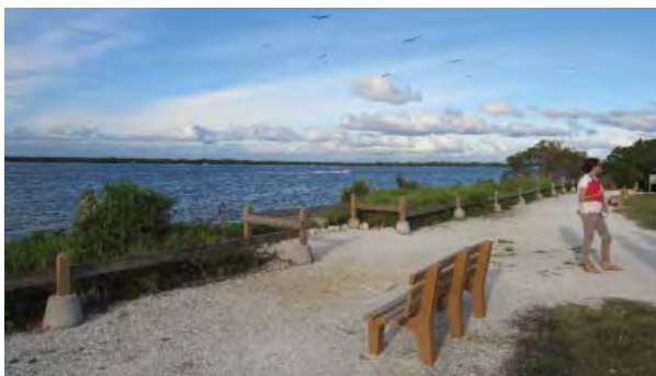
FIGURE 3-160. Board fence on site-cast, moveable footings; view east at beach berm.
