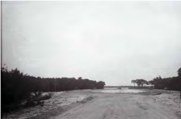
FIGURE 2-43. View north into parking area, filling and grading in progress, 1950. (DESO Archives)
