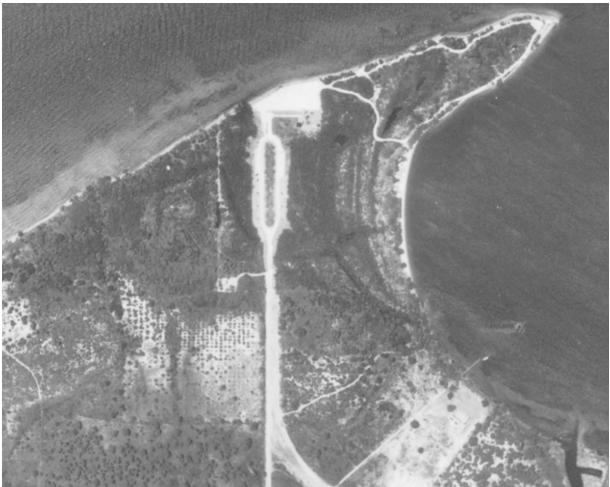
FIGURE 2-52. Aerial photo, U.S. Agriculture Soil Conservation Service, 1951. Construction appears essentially complete, including the parking area, walks, plaza, contact station, and freshly filled trails. (TRS Environmental and Historical Research, Inc. See also Appendix C)
