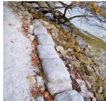
FIGURE 3-182. Revetment further south on cove trail, view north.
