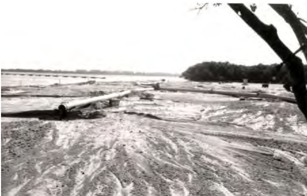
FIGURE 2-75. Hydraulic filling for major beach re-nourishment, plaza beach and north shore, 1961. (DESO Archives)
