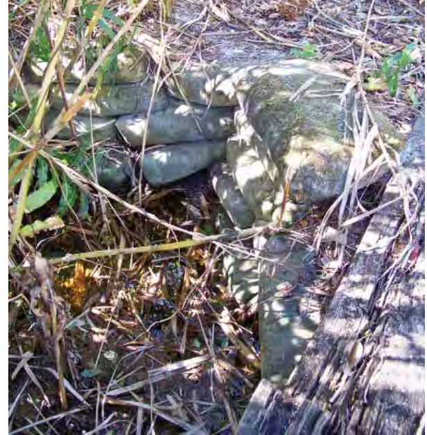
FIGURE 3-40. Culvert/headwall, south side of maintenance drive, view west.
