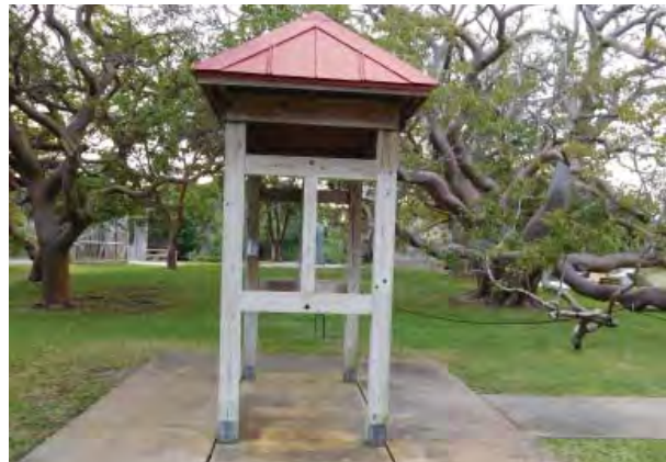
FIGURE 3-143. Kiosk, view west..
