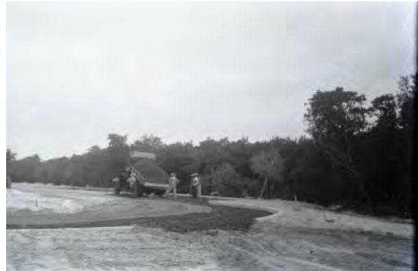
FIGURE 2-44. View south into parking area, paving in progress, 1950. (DESO Archives)
