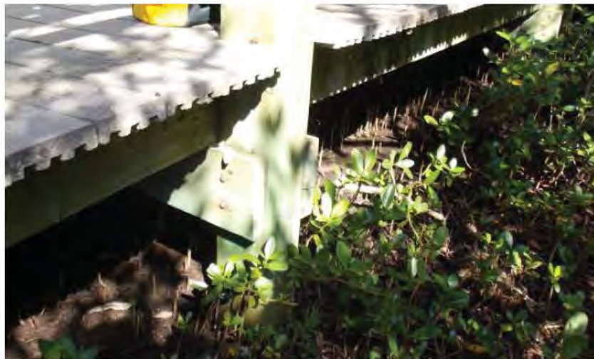
Photo 2; View of typical connection of 2x8 girders to 6x6 wood post.
