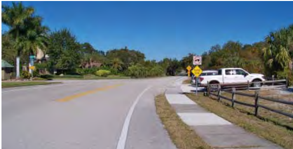
FIGURE 3-3. Approach to the Memorial site (view north).
