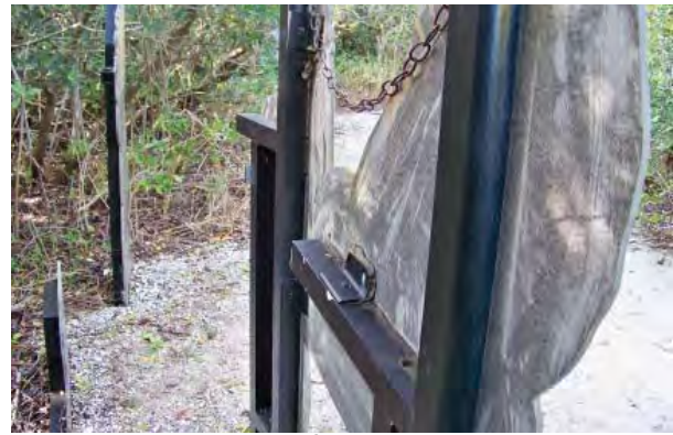
FIGURE 3-148. Detail of panels seen in Figure 3-147. (South loop trail, view west.)
