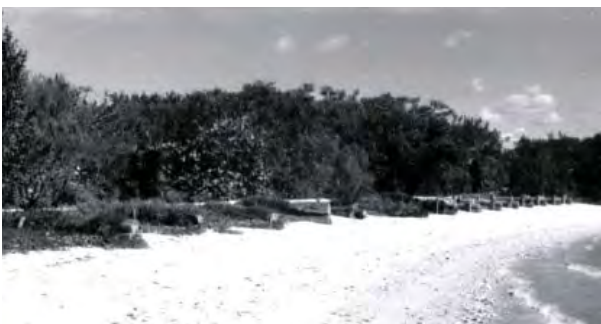
FIGURE 2-69. Cypress log groins along cove trail, installed after earlier palm logs failed, 1959. (DESO Archives)
