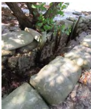
FIGURE 3-178. Channel seen in Figure 3-177, view west-northwest.
