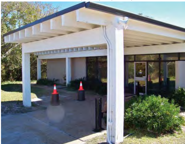
FIGURE 3-106. Visitor center north facade, view southeast.
