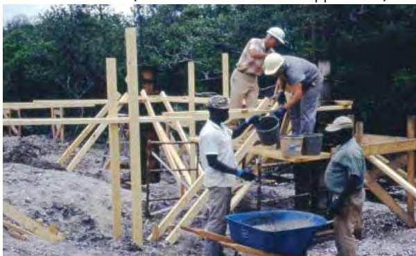
FIGURE 2-90. Visitor center construction, 1967-1968; forming and pouring concrete columns and beams. (DESO Archives)
