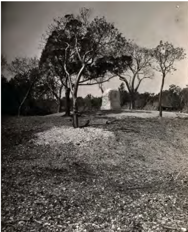
FIGURE 4-10. View of the monument and surrounding gumbo limbo grove, 1939. (DESO Archives)
