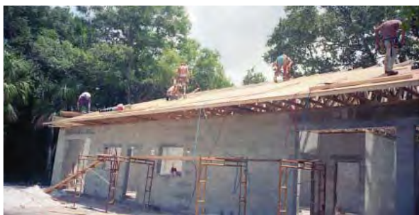
FIGURE 2-100. Maintenance building construction, 1994; view south. (DESO Archives)
