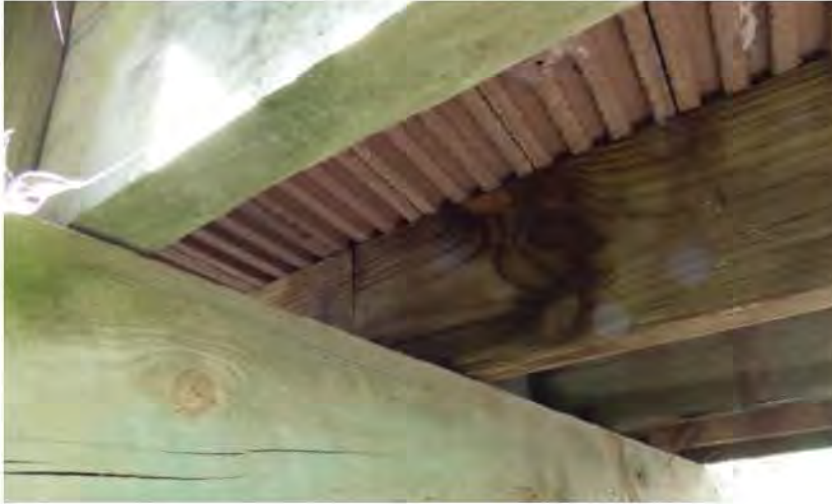
Photo 3; Typical view of floor joists bearing on wood girder.
