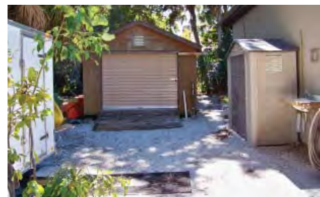
FIGURE 3-132. View south to storage sheds east of administration/maintenance.
