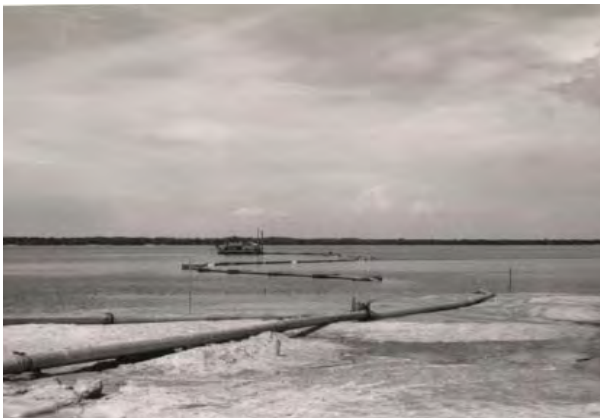
FIGURE 2-74. Hydraulic filling for major beach re-nourishment, plaza beach and north shore, 1961. (DESO Archives)
