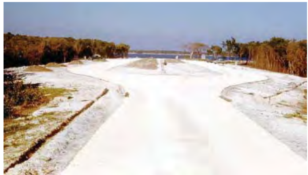
FIGURE 2-46. View north into parking area, paving appears complete, topsoil delivered, 1950. (DESO Archives)
