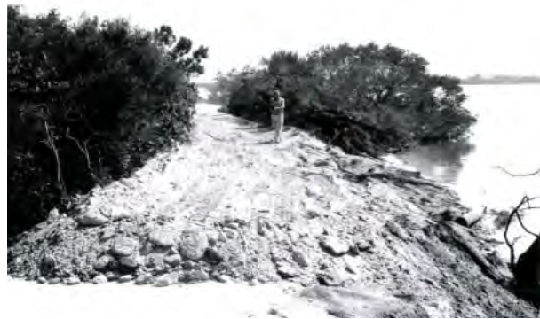
FIGURE 2-72. Post-Donna repairs in progress, north shore trail, April 1961. (DESO Archives)
