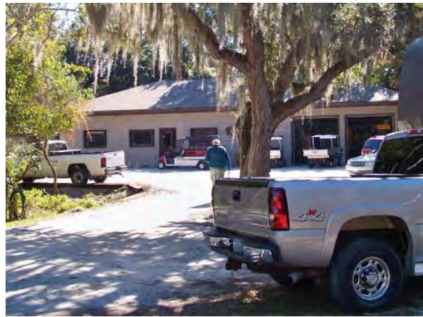
FIGURE 3-127. Administration/maintenance: view south to main facade.
