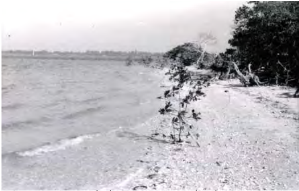
FIGURE 2-73. North shore mangrove plantings, January 1961. (DESO Archives)
