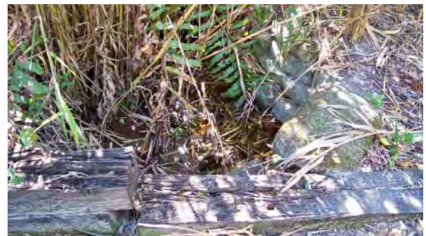
FIGURE 3-174. Channel at midpoint of maintenance drive, view south.
