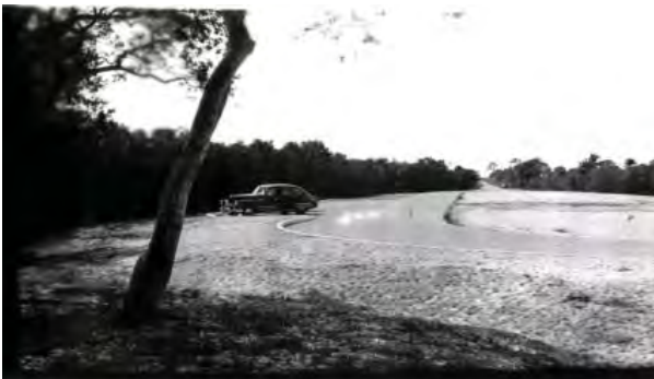
FIGURE 2-45. View south into parking area, paving appears complete, 1950. (DESO Archives)
