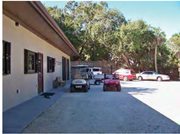
FIGURE 3-128. Administration/maintenance: view west, just in front of building.
