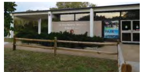
FIGURE 3-107. Exterior circulation at west facade.
