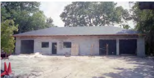
FIGURE 2-101. Maintenance building construction, 1994; view south. (DESO Archives)
