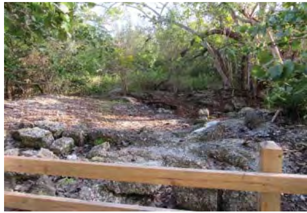
FIGURE 3-98. View south, along the structure's west edge.
