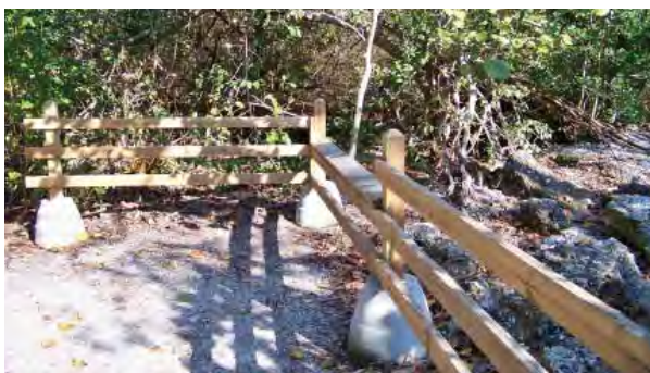
FIGURE 3-161. Board fence on moveable footings, view east at tabby house ruin.
