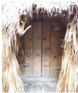
FIGURE 3-116. Detail of storage shed.
