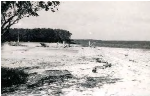
FIGURE 2-71. Hurricane Donna damage, 1960; the Superintendent's Monthly Report described this photograph as showing the area "pushed back 20' to 30', waves are now eating into grass at right of flagpole." (DESO Archives)
