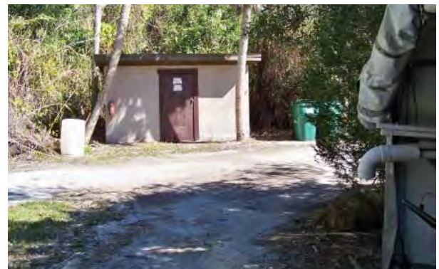
FIGURE 3-136. Hazardous materials storage building, view east from north end of quonset hut.
