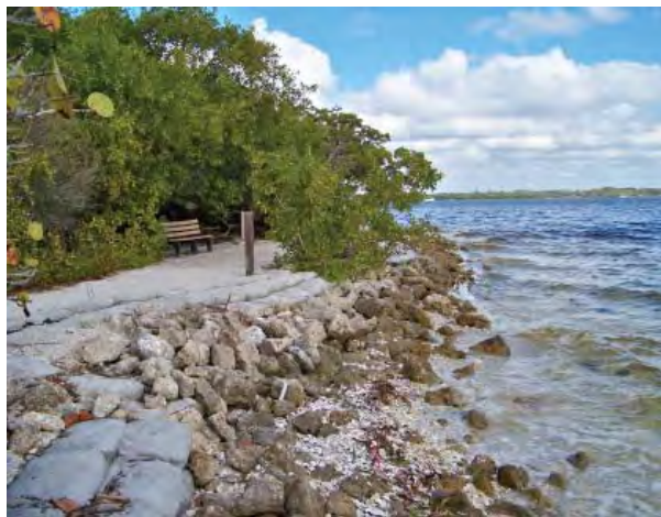
FIGURE 3-45. Cove shoreline south of point, view north.
