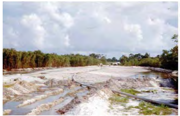
FIGURE 2-42. View south into parking area, hydraulic filling in progress, 1950. (DESO Archives)
