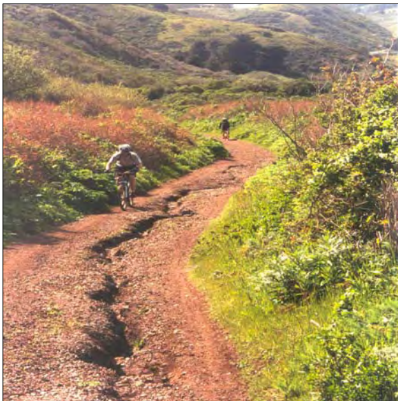
Photo 1.13 Severe trail erosion on Julian Road.
