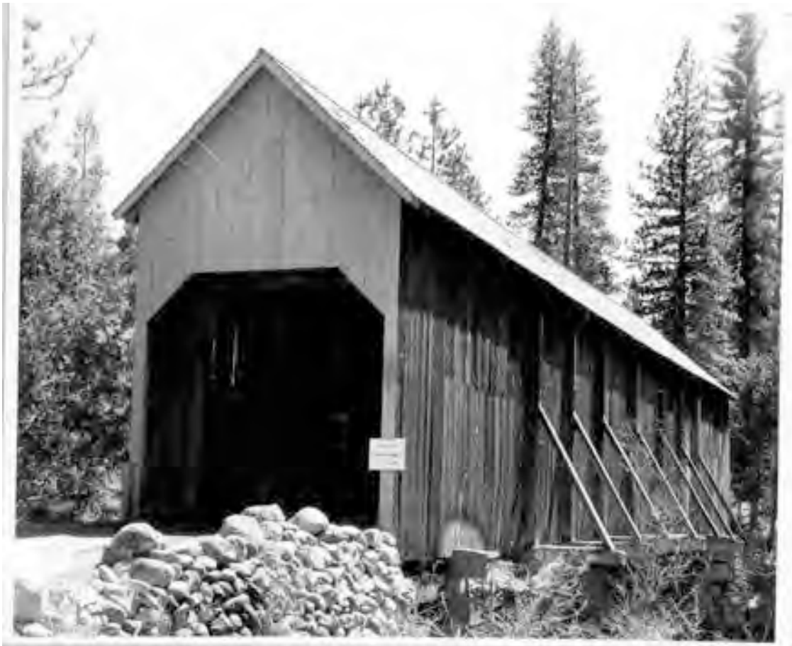
PHOTO 5-1: WAWONA COVERED BRIDGE 1957 (NPS 1957)
