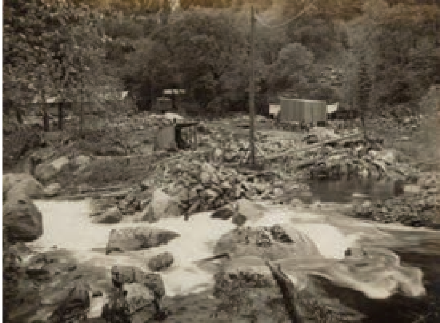
PHOTO 4-13: BEFORE CASCADES DIVERSION DAM CONSTRUCTION (FROM SOUTH BANK)-UNDATED (TAKEN CIRCA 1916 OR 1917, IMMEDIATELY PRIOR TO DAM CONSTRUCTION) (NPS UNDATED)
