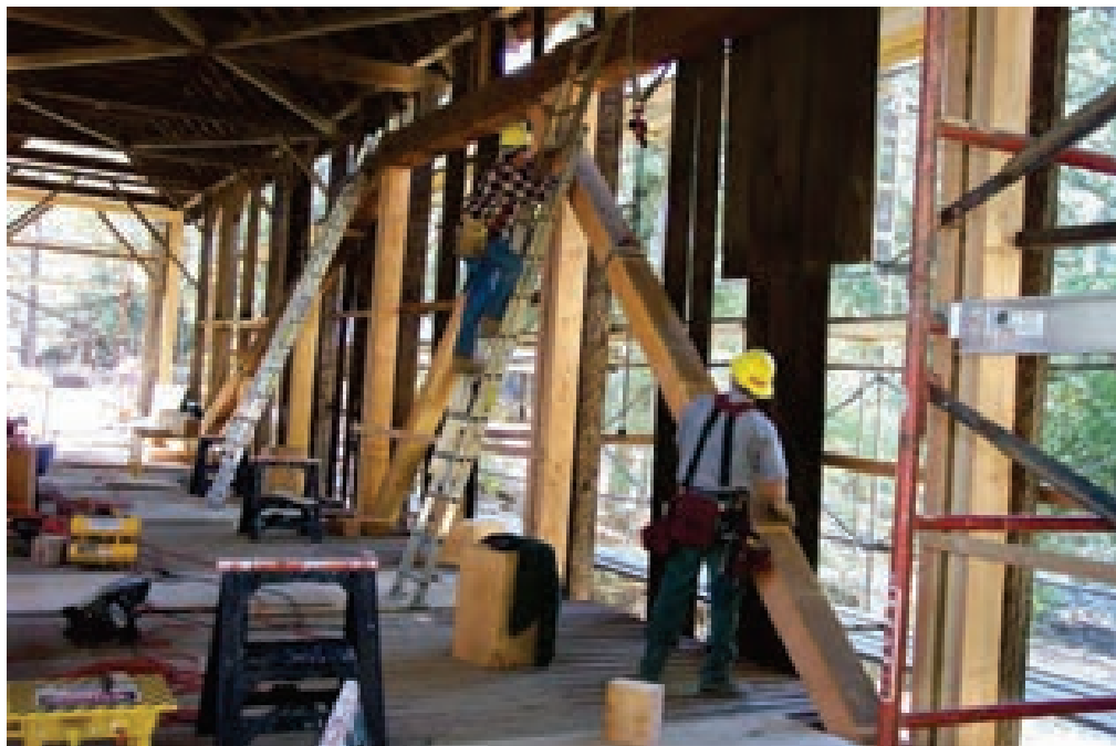
PHOTO 5-2: WAWONA COVERED BRIDGE 2005 (NPS 2005)
