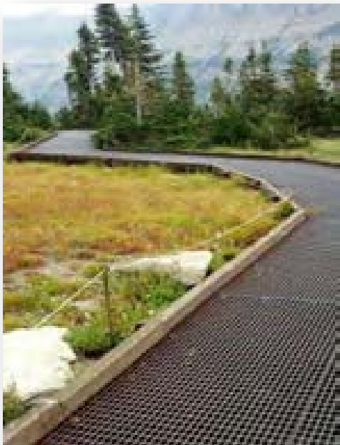
Figure 3-7 and 3-8: Metal grate boardwalk in Glacier National Park
