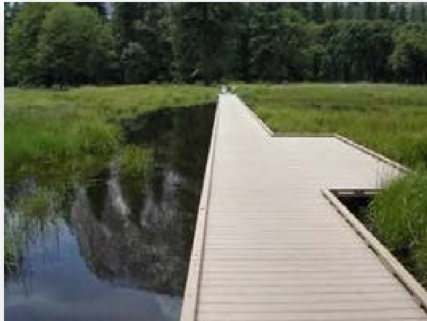
Figure 3-1: Cook's Meadow boardwalk in Yosemite Valley. Constructed of recycled plastic, a material commonly used in Yellowstone National Park, where a roughened surface is used to provide traction on frosty mornings. However, Yosemite managers have found that this product does not last and requires frequent maintenance.
