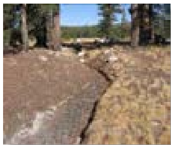
Fig. 1-11. Ditch draining kettle pond
