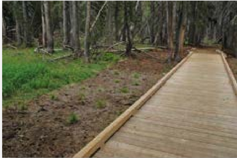
Figure 3-2: Newly installed TimberSIL® boardwalk at Tenaya Lake 2012
