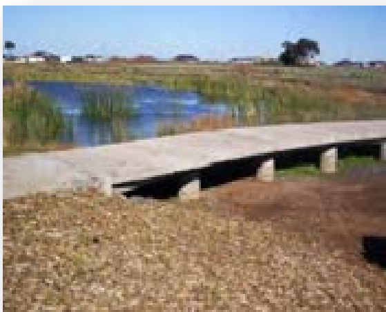
Figure 3-3: Boardwalk Estate, Melbourne Australia: Permatrak® boardwalk with pier supports allows water flow underneath the structure
