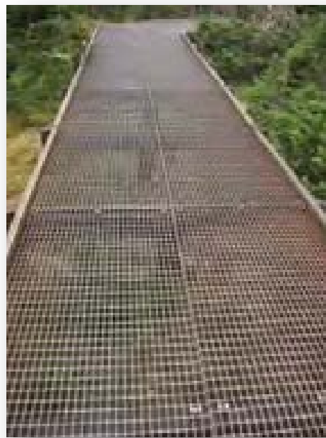
Figure 3-7 and 3-8: Metal grate boardwalk in Glacier National Park
