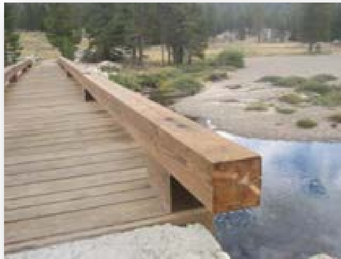
Figure 3-12: Bridge over the Tuolumne River
