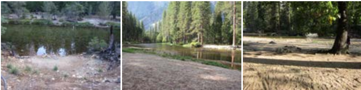
Figure 7: Use of the riverbank at the current river access in Lower Pines Campground has caused vegetation trampling and heavy erosion of this highly susceptible riverbank (left). Use will instead be directed to resilient sandbars such as these, located a short walk downstream (middle and right).
