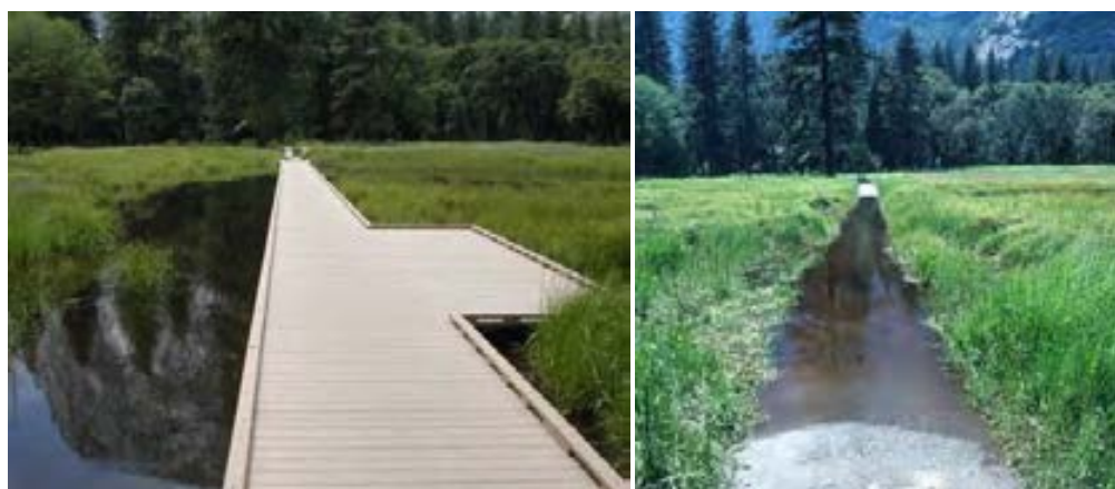
Figure 17: Trails through frequently inundated wet meadows, such as in cook's meadow pre-restoration (left), cause peripher vegetation trampling and soil compaction and make access difficult. A boardwalk installed in 2005 allows for visitor access into the meadow environment and protects the meadow soils and hydrology.
