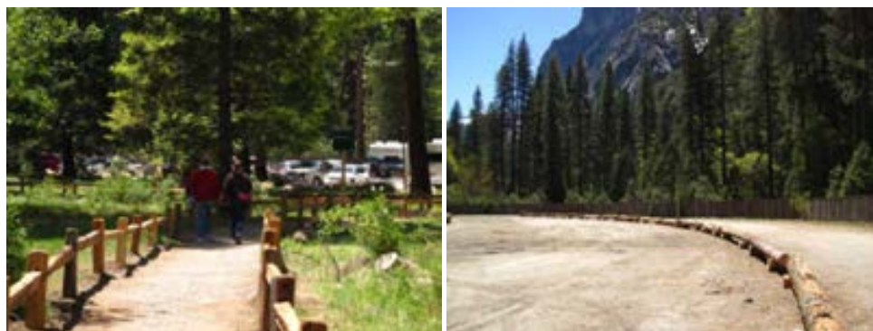
Figure 13: Post and rail fencing (Left) and log and block fencing (right).
