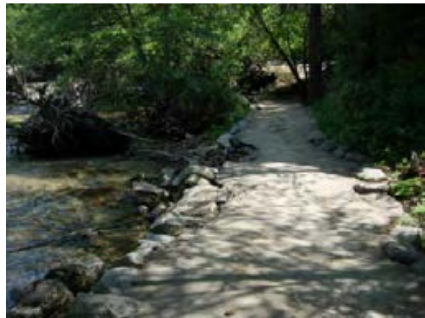
Figure 2: Stock trail in Happy Isles reach passes through riparian habitat. Its hardened surface affects natural hydrologic processes by preventing sediment transport and capture.
