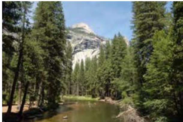
Figure H-25: Stoneman Bridge. NPS 2012
