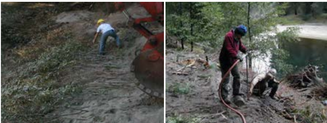
Figure 15: Yosemite restoration staff have employed bioengineering techniques in past park projects including Brush layering with willows (left). Restoration workers insert live willow cuttings with the aid of a hydrodrill to revegetate this riverbank (right).
