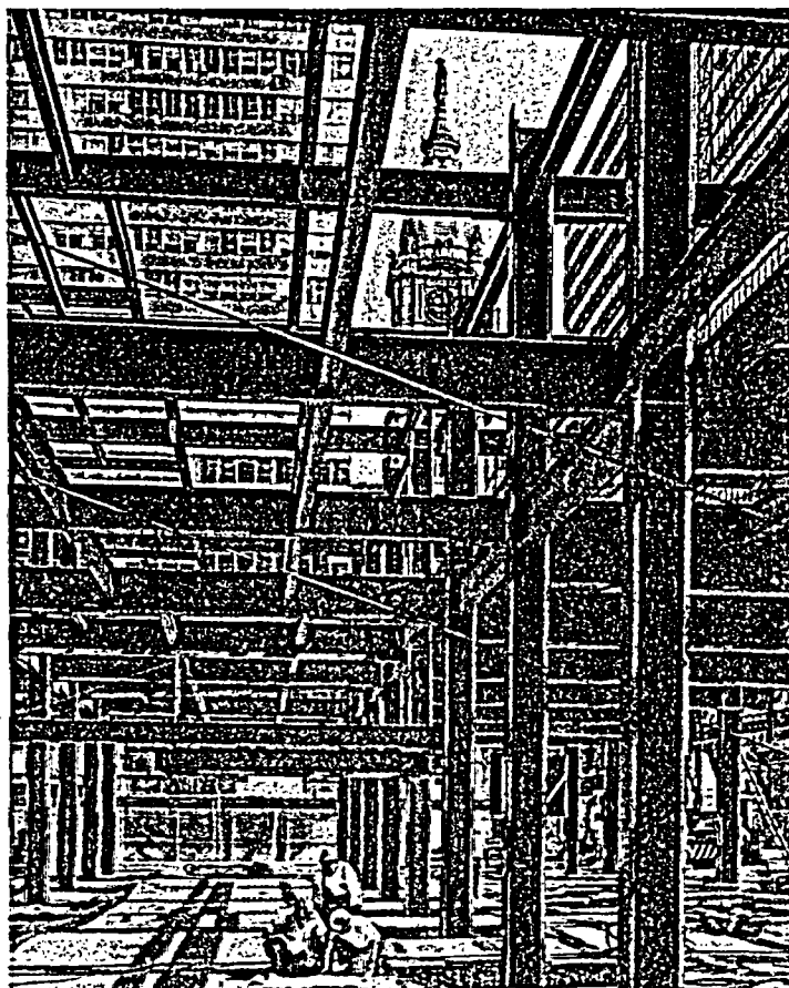
PENN CENTER CONSTRUCTION CONTINUES
