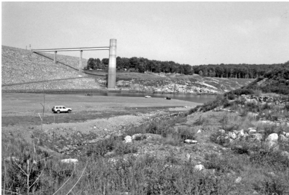
Figure 5. View of the Francis E. Walter Dam from the left (south) abutment, showing rip-rap lined earthen banks, control tower for outlet conduit, and ledges of Mississippian-age Pocono sandstone in pool area to right.
