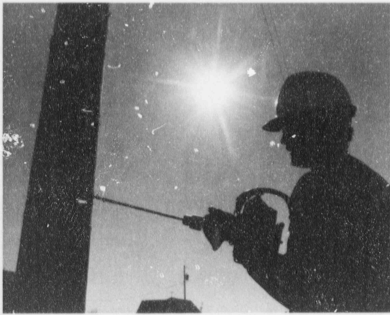
Supplemental treatments of our wood poles with preservatives should extend their life by ten years or more and save about $10 million in pole replacements.
