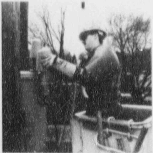
Electric Operations personnel keep busy throughout the year maintaining OPPD lines. Here, an OPPD line technician replaces a squirrel guard.
