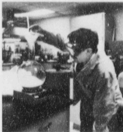
A North Omaha Station lab employee weighs disodium phosphate which is added to boiler water to maintain boiler efficiency and cleanliness.
