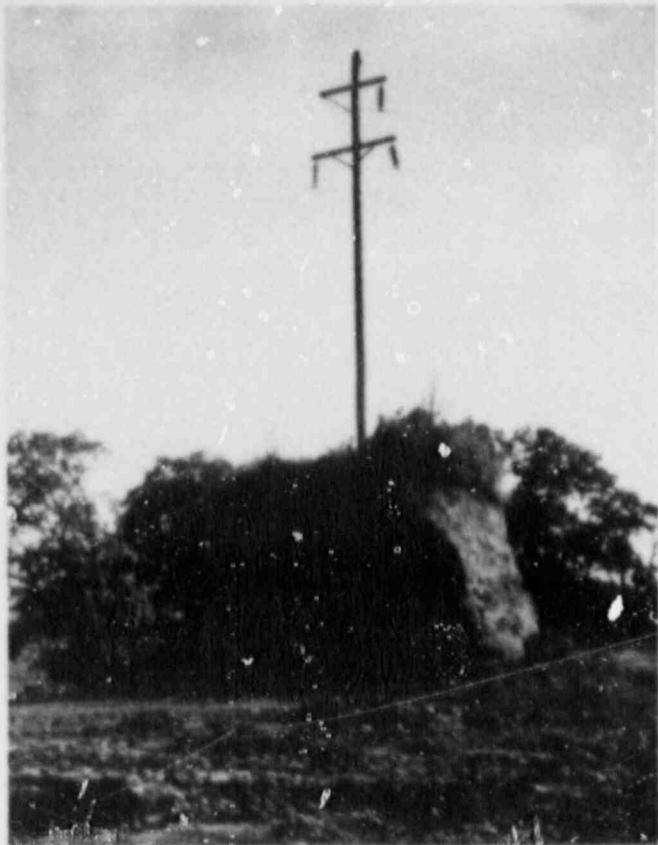
WIPCO crews had to move a pole on the East Hannibal transmission line to accommodate construction of the Central Illinois Expressway near East Hannibal.
