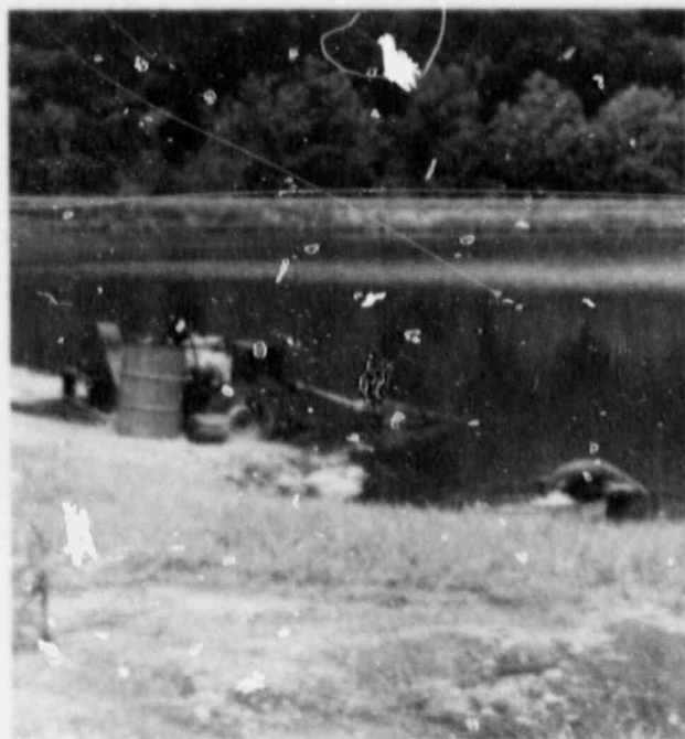
Pearl's ash pond was pumped and excavated in 1987. Under normal operating procedures in the past, the pond has had to be excavated about every four years.
