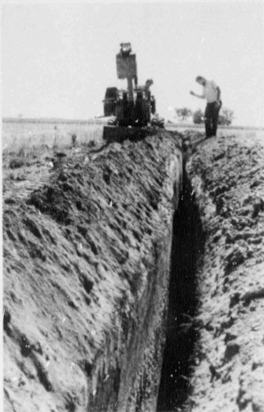
Pictured above is the installation of a horizontal loop for a ground-source heat pump. Piping is installed in trenches at depths of three and five feet.
