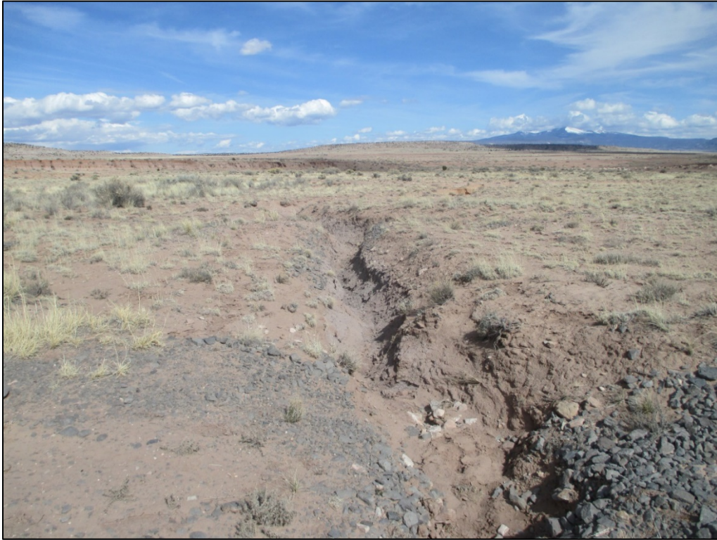
PL-1. Erosion of the Site Perimeter Road (South Area)
