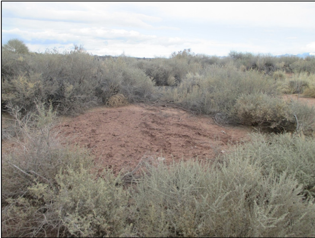
PL-13. Area of Depression Repaired in the Asbestos Disposal Area
