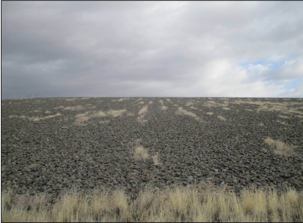
PL-9. South Side Slope of the Main Tailings Disposal Cell
