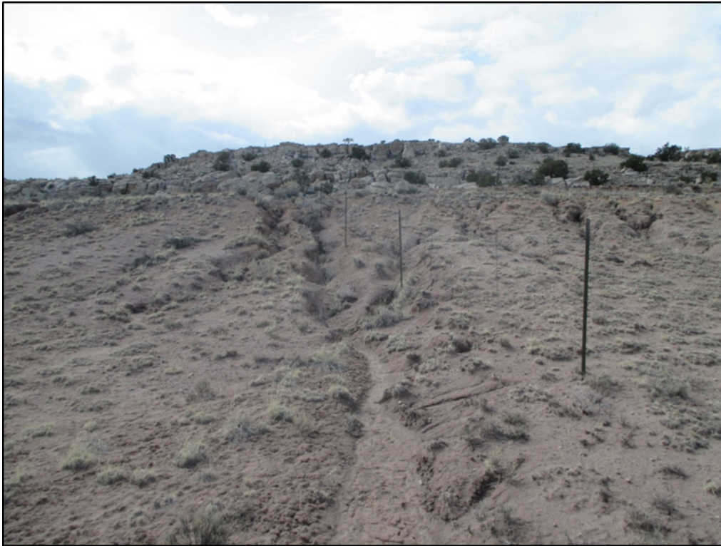
PL-3. Erosion Along the Perimeter Fence
