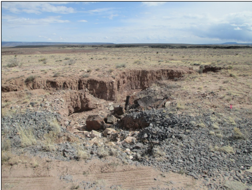
PL-2. Erosion Near the Site Perimeter Road (North Area)
