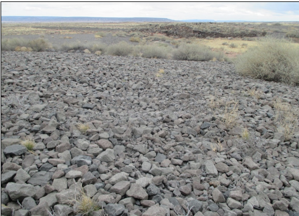
PL-14. Minor Depression on the Asbestos Disposal Area North Side Slope
