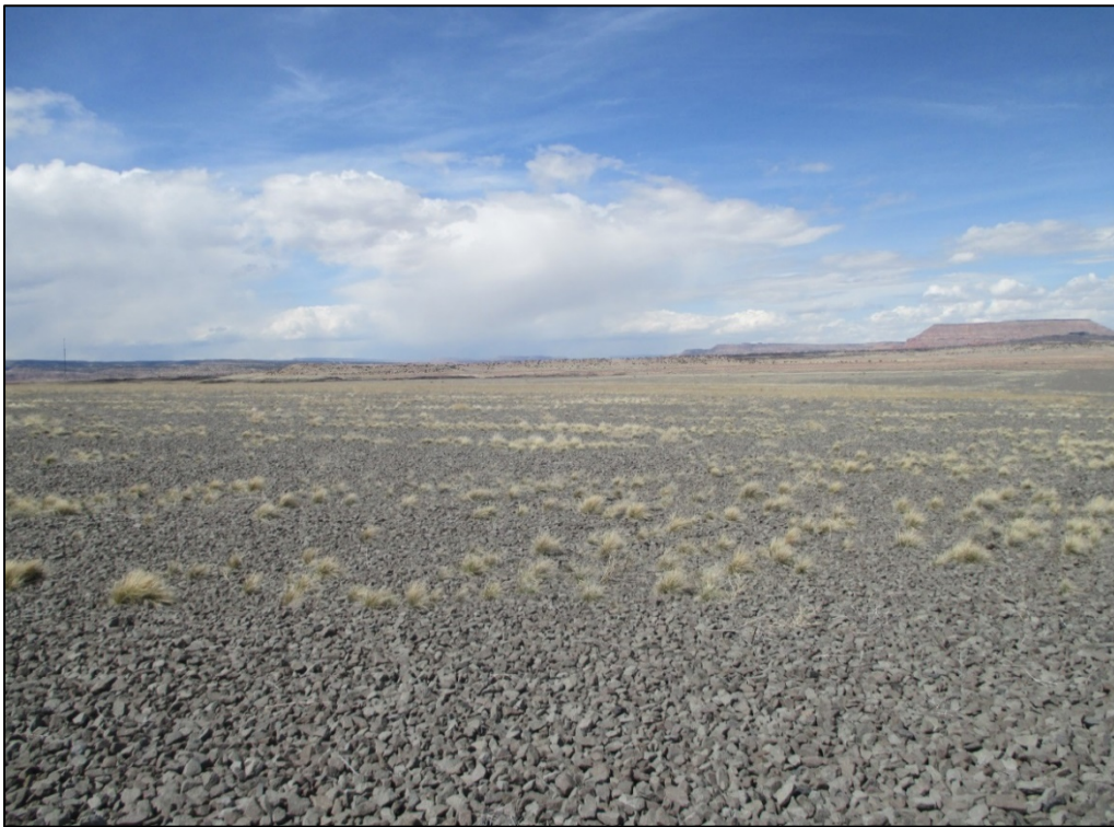
PL-6. Top Slope of the Main Tailings Disposal Cell
