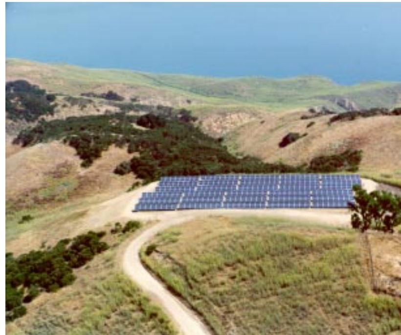
ETS staff managed this PV installation off the California coast on Santa Cruz Island. This 130 kW site validates the cost-effectiveness of renewable technologies in isolated, remote applications.
