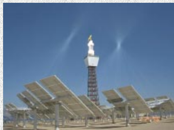
Solar Two at Daggett, California
