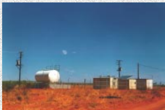
Eppennara power station
