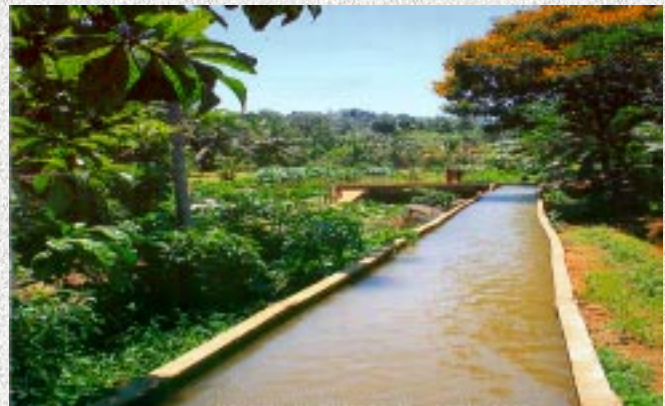
Micro-hydro electric power station provides clean, safe energy in Sri Lanka.
