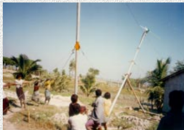
Installation of 1.5-kW wind turbine in Chokaria, Bangladesh
