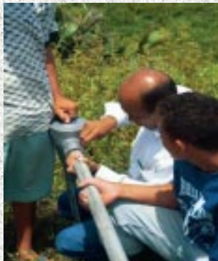
Installation of REGAE financed wind-electric water pumping system
