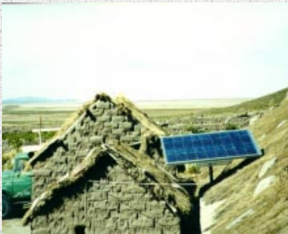
Typical solar home system installed in the altiplano
