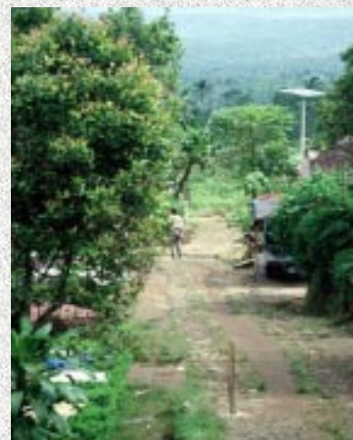
Individual PV home system
