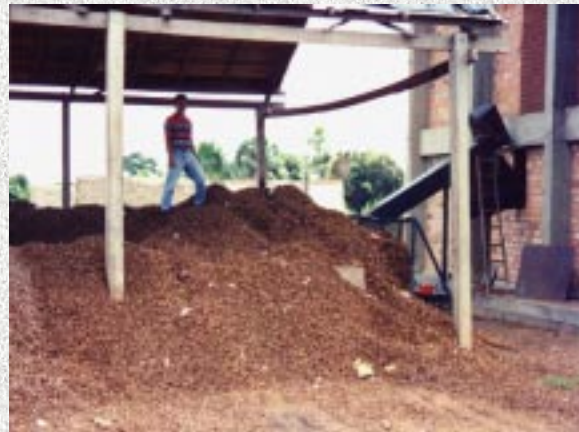
Riberalta biomass 1-MW power plant
