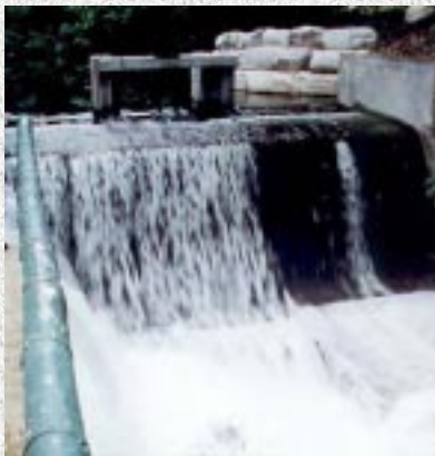
A view of the micro-hydro plant
