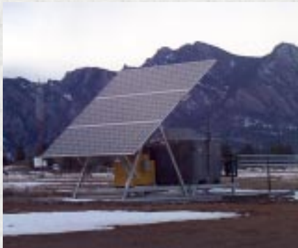
SunWize Wind-PV-Diesel system at the National Wind Technology Center
