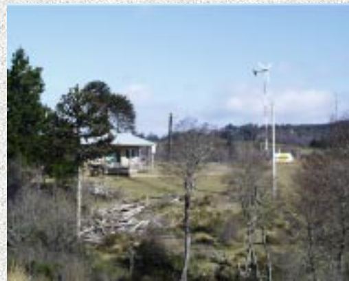
Village of Villa Las Araucarias and the installed power system
