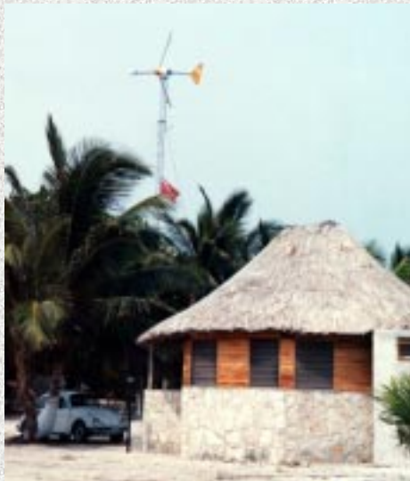
Costa de Cocos 11-kW wind-diesel hybrid system
