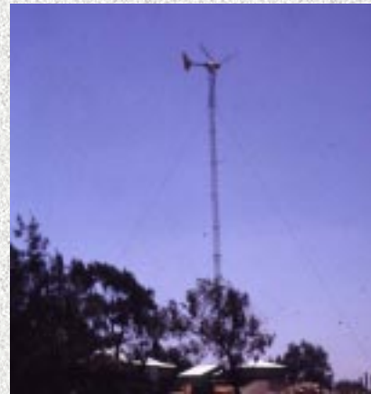
Wind hybrid power system in West Timor
