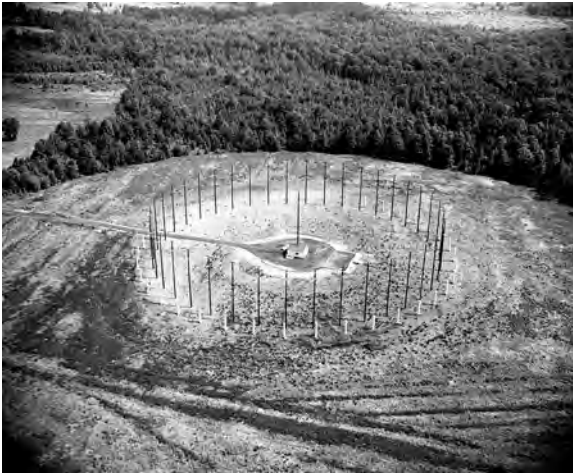
Huff-Duff. Known formally as a Wide-Aperture Circularly Disposed High Frequency Radio Direction Finder, this array of antennas and processing equipment in the central building is capable of identifying the direction from which high-frequency radio signals are emanating. This array, used by NRL in the late 1950s and 1960s, was located at Hybla Valley, Virginia, not far from Washington, DC. (NRL photo 58-039971.jpg, 58-040249.jpg, or 60-45951(1).jpg)
