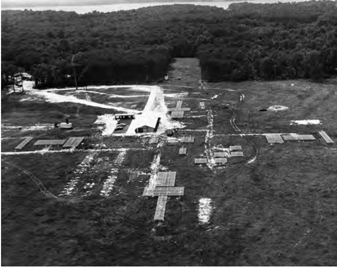
Minitrack Footprint. A pivotal component of Project Vanguard, the satellite-tracking system called Minitrack would become the prototype of the nation's primary satellite tracking system, NAVSPASUR, in the early years of the Space Age. This 1956 photo shows the primary site of the Minitrack system in Blossom Point, Maryland. (NRL photo 56-045950.jpg)
