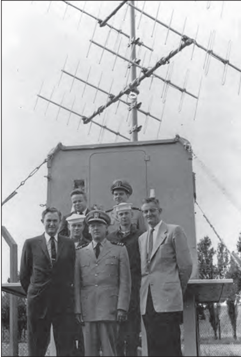
The Huts. An important part of the world's first ELINT spy satellite system were portable command, control, and listening huts placed around the periphery of the Soviet Union and elsewhere by which operators could communicate with GRAB satellites as they passed overhead. Included in this photo are Countermeasures Branch Head Howard Lorenzen (leftmost on bottom), GRAB Project Engineer Reid Mayo (leftmost at top), hut operators in the sailor hats, two officers, and Radio Control Hut Engineer William Edgar Withrow (rightmost at bottom). ( NRL photo Radio.tif )
