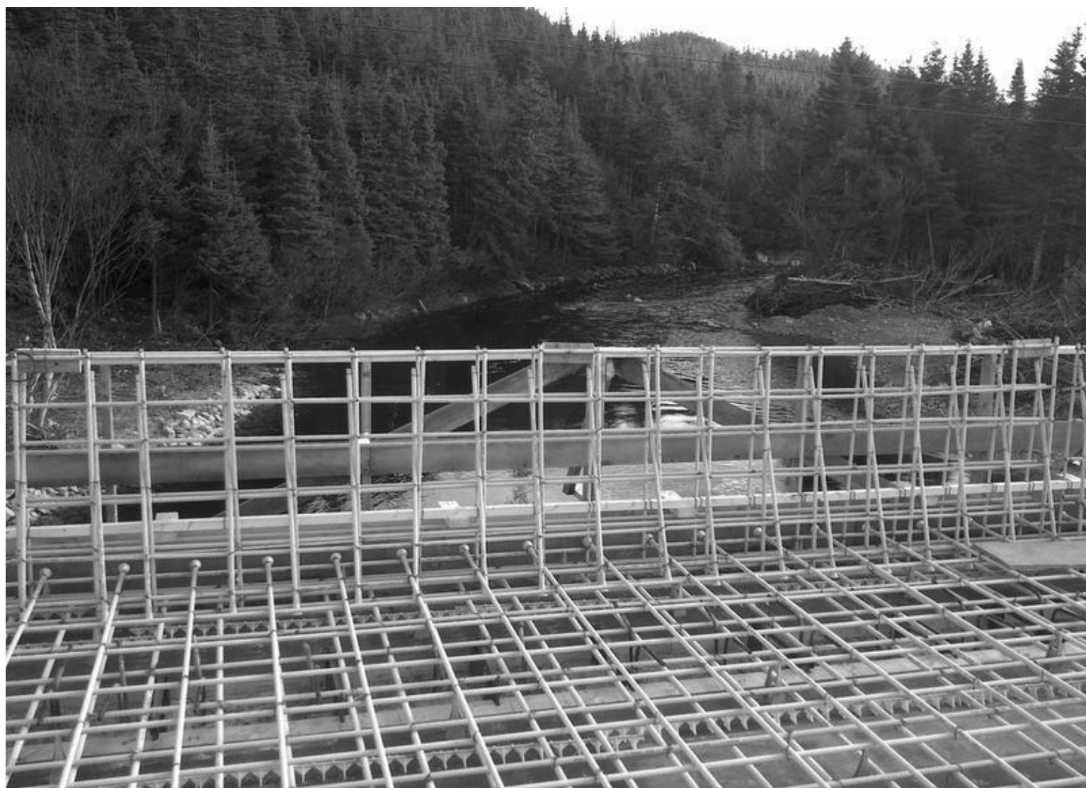
The reinforced polymer mesh is strong and lightweight, non-corrosive and relatively inexpensive. It's also starting to come into wide use in the province where it was first developed. CONTRIBUTED/NSRBA
