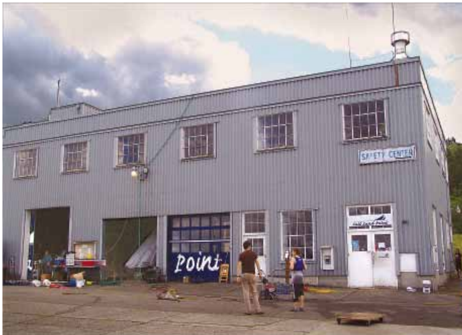
Photo above - The famed Building 11 as mentioned in this article with the entrance into Sail Sand Point headquarters.
