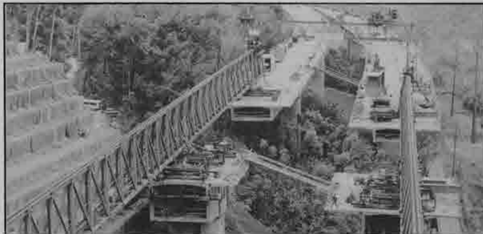
Above: A crawling gantry truss hydraulically transports pre-cast segments into place.
