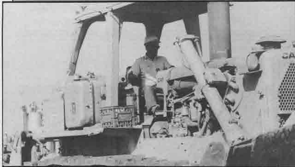
Above: Dozer operator Glenn Harman.
