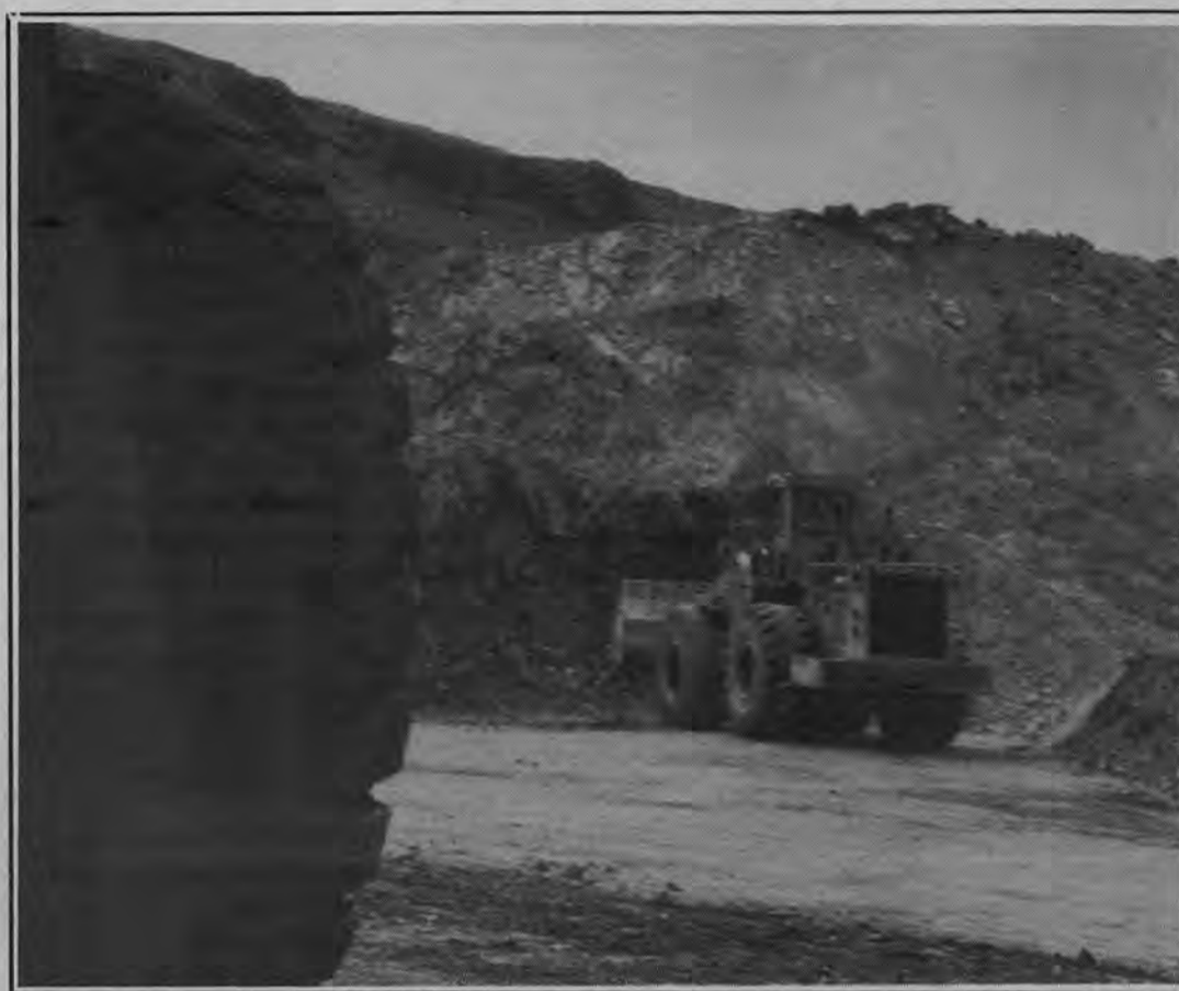
Huge tires from Haulpak truck appear to dwarf Cat loader working at Rain Pit.
