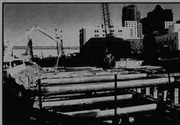
Tubular struts for soil stabilization are visible along the cut-and-cover section.
