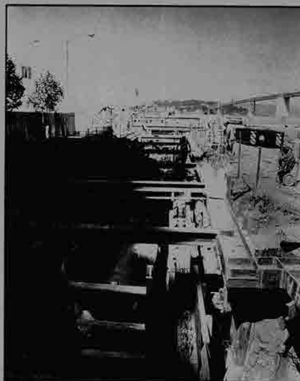
The new Howard Street sewer outfall takes shape.
