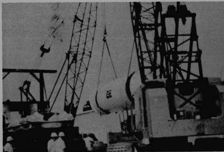
PICTURED TOP LEFT at the nuclear plant site in Florida, is a 600-ton steam power generator fastened to Bigge's lifting gantry. At top right, the 800-ton nuclear reactor core sits on the jacking frame. It takes two cranes working together (bottom left) to lift the 350-ton
