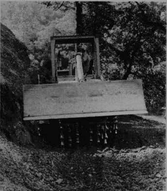
Bob Molini runs compactor for C.R. Fedrick on Unit #14.
