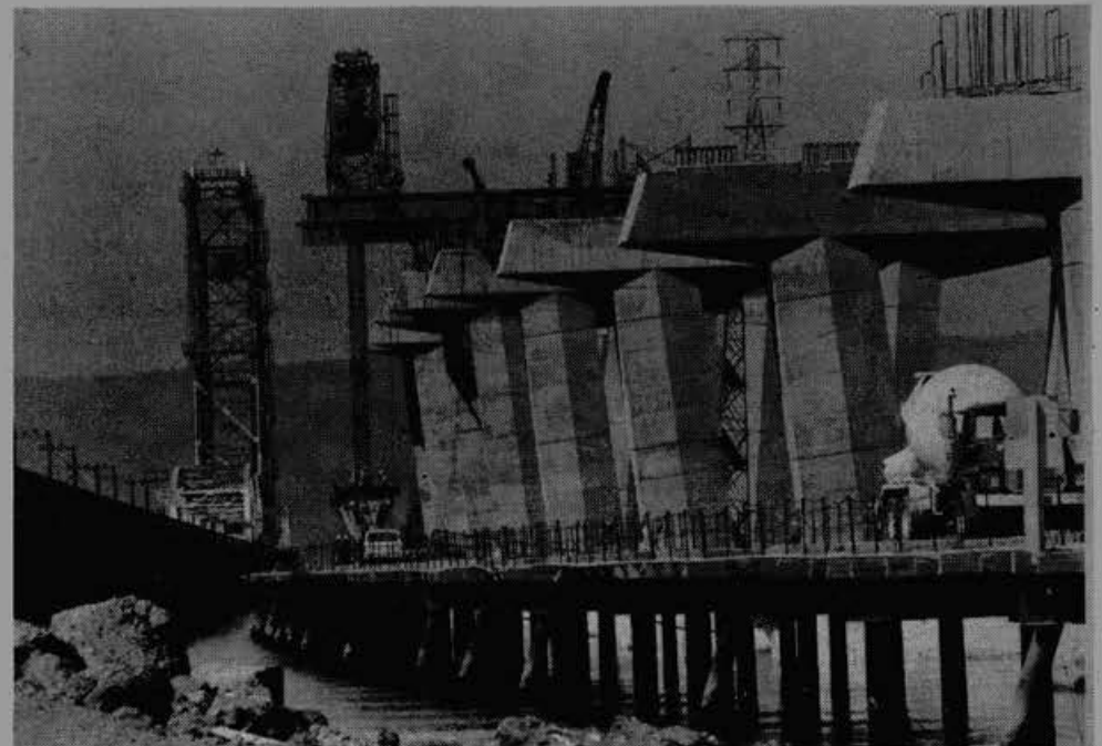
Using unique overhead crane make progress on Guy F. Atkinson's arrangement, work continues to Dumbarton Bridge Job.
