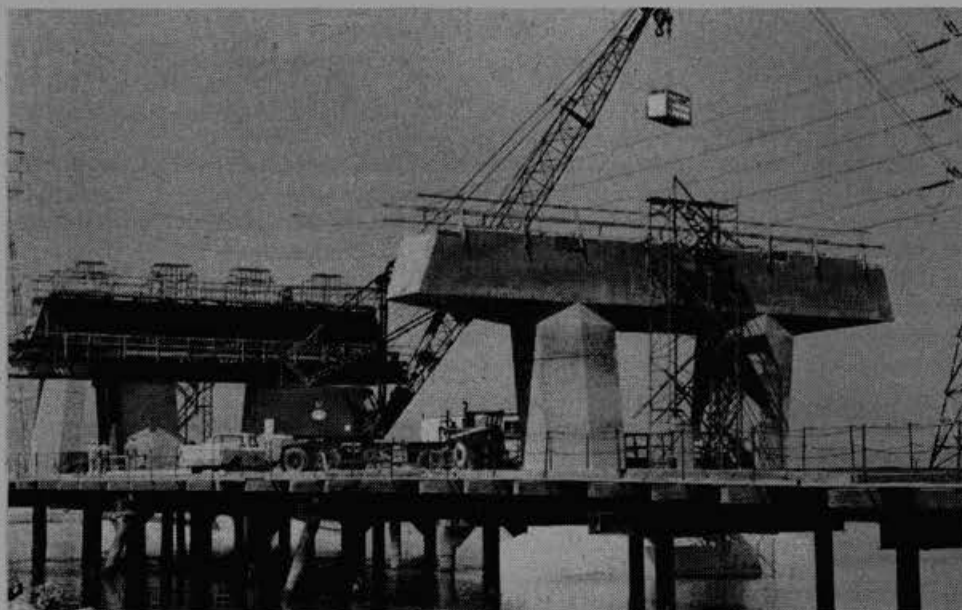
Using unique overhead crane make progress on Guy F. Atkinson's arrangement, work continues to Dumbarton Bridge Job.
