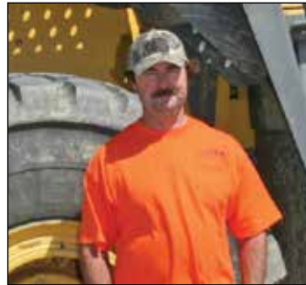
Loader Operator Gary Davis moves native fill to Sherman Island for Asta Construction.
