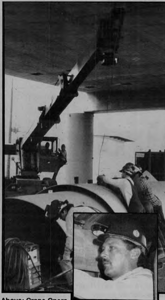
Above: Crane Operator Joe Wint lifts steel jackets into place while ironworkers weld them together. Inset: Crane Operator Joe Wint.
