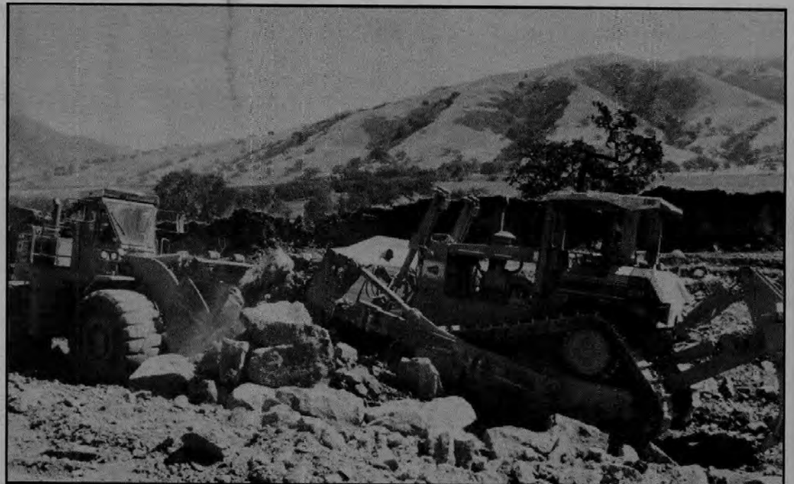
Below: 20,000 tons of rocks are removed and stored during excavation of the three major road cuts.
