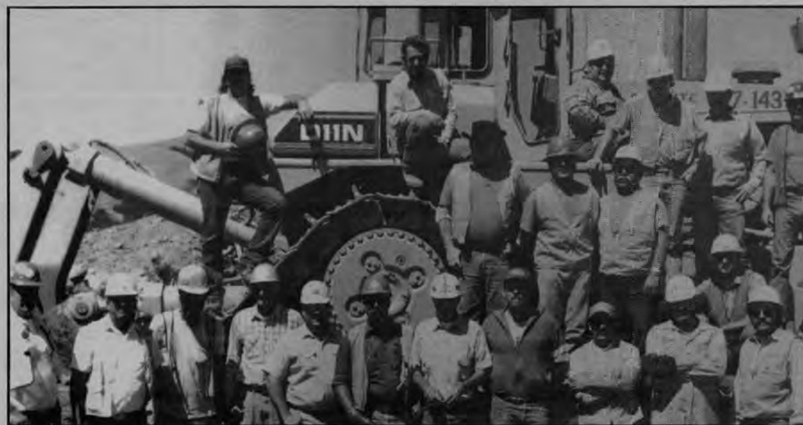
Granite's crew at Pacheco Pass Hwy. project.
