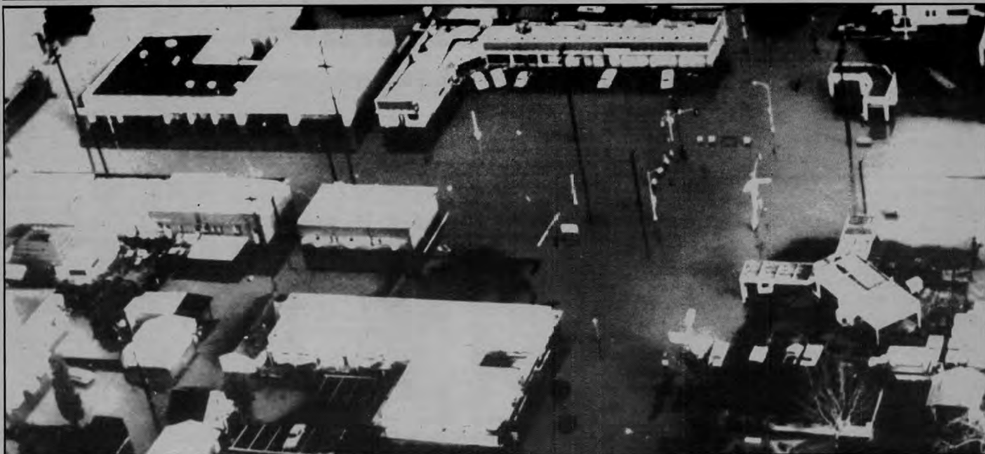
Heavy rains in 1969 inundated downtown Fresno, prompting officials to develop a rural flood control system, which Operating Engineers have been working on for the past several years.
