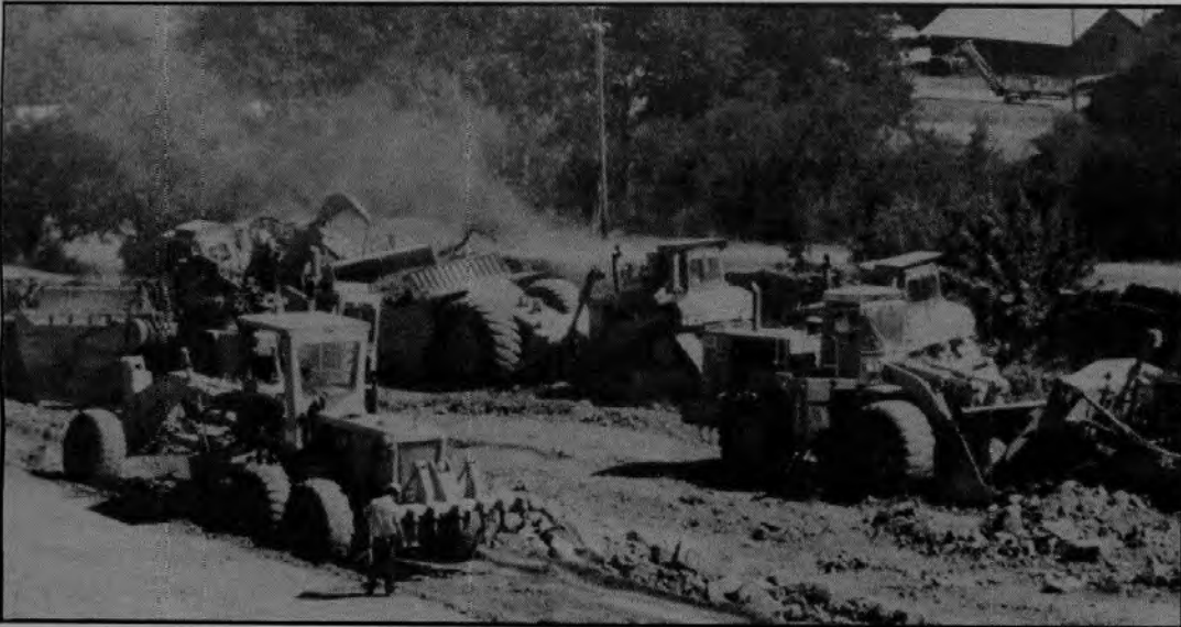
Top: The largest of the road cuts requires 300,000 yards of excavation.
