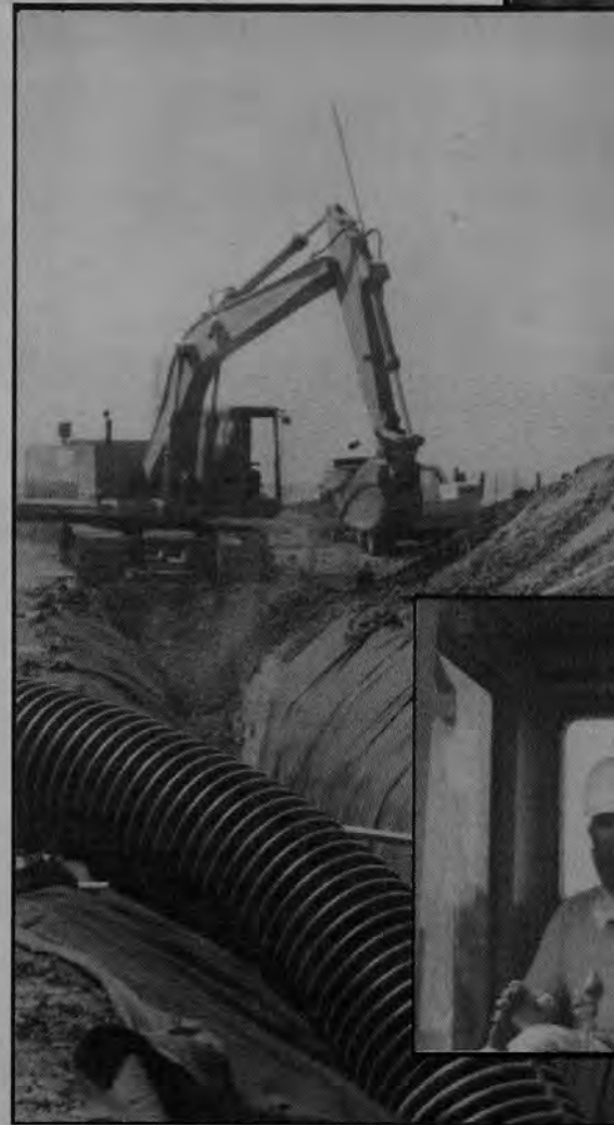
Right: The dam's spillway under construction in August.
