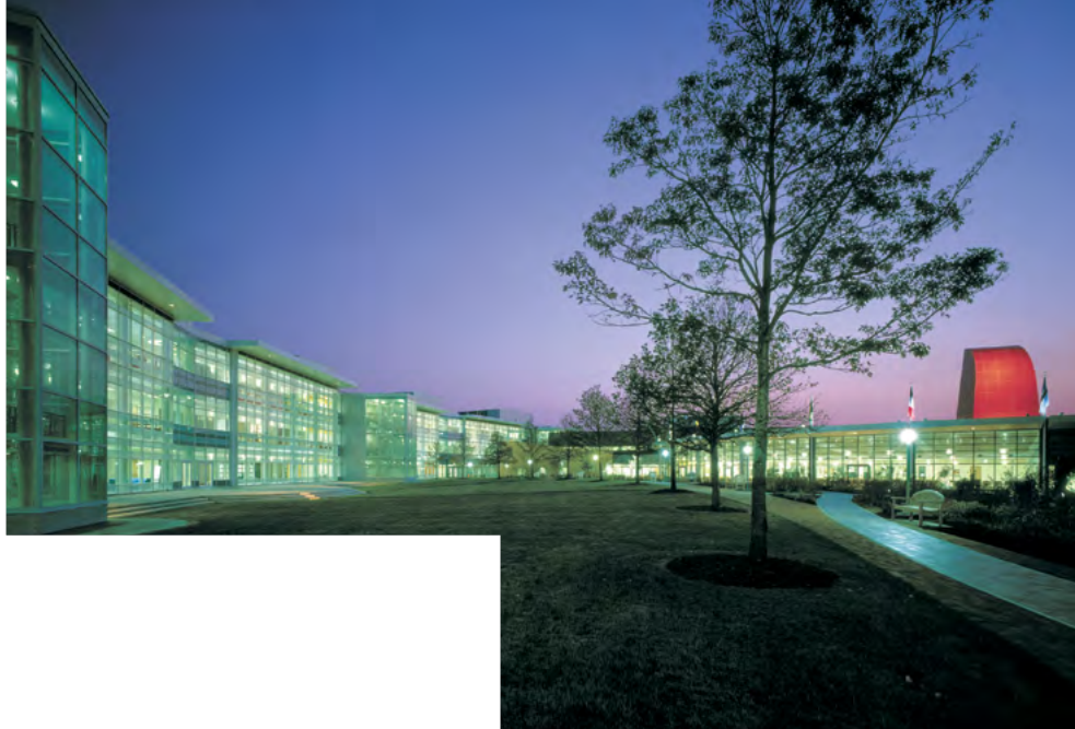
Photo: Owens Corning World Headquarters, Toledo, OH
