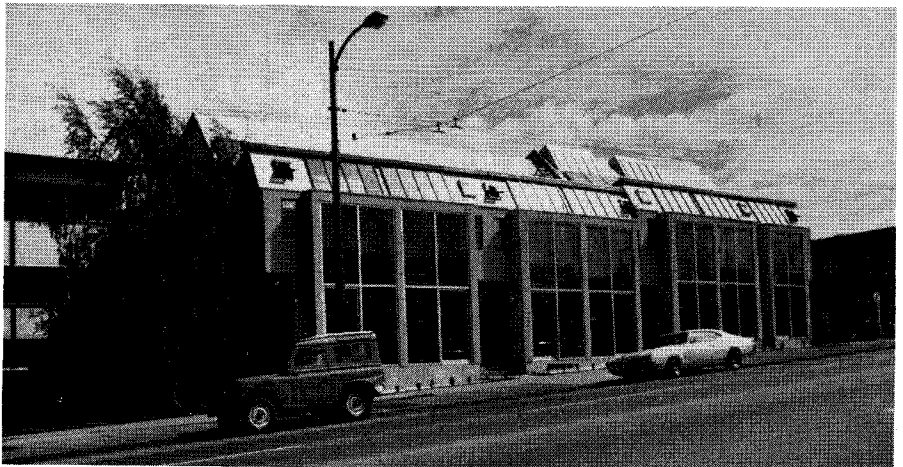
Fig. 13. South side of Vancouver townhouse building (see section above).
