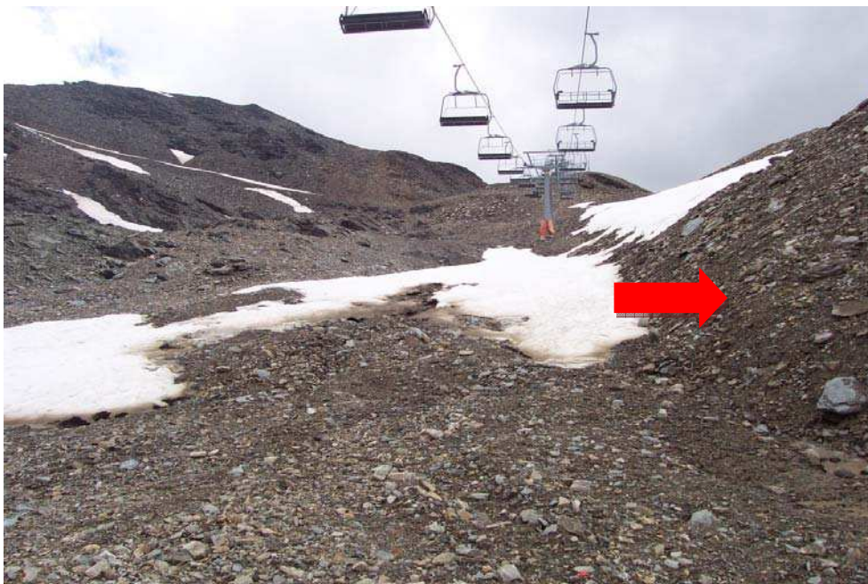
Fig. 9 – Photograph of the debris ridge along the ski lift "Madritschjoch" in July 2006. Photograph by A. Zischg. The red arrow shows the location with of the observed slope deformation.
