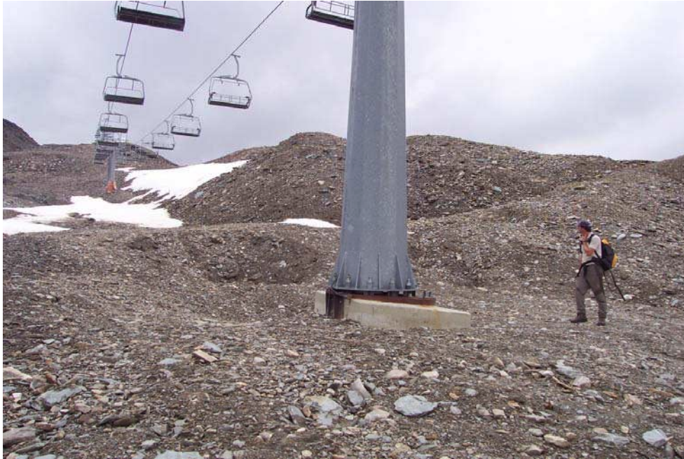
Fig. 8 – Photograph of the re-adjustment of the position of the pillar no. 12 of the ski lift "Madritschjoch". Photograph by A. Zischg.
