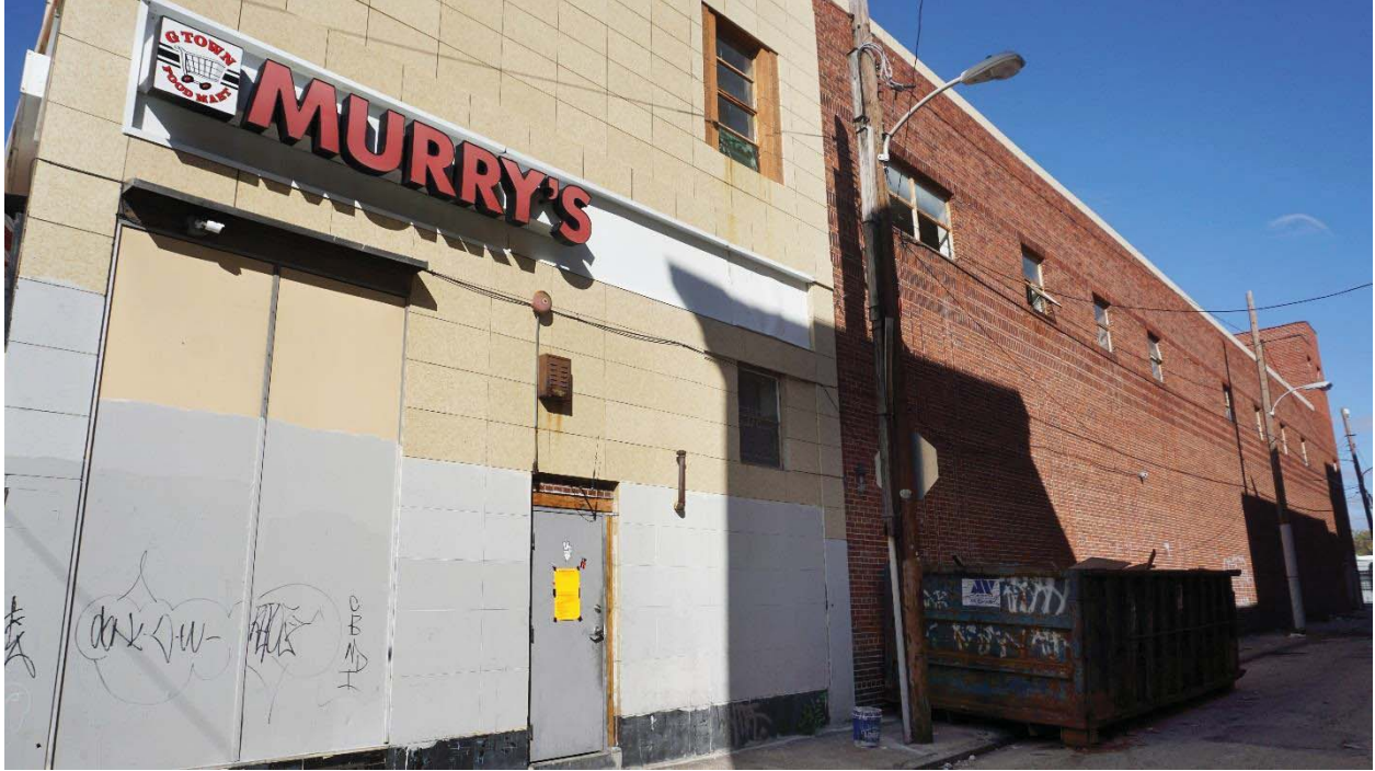
Figure 6 View of the building's Southeast façade. November 2019. Photo by Author.
