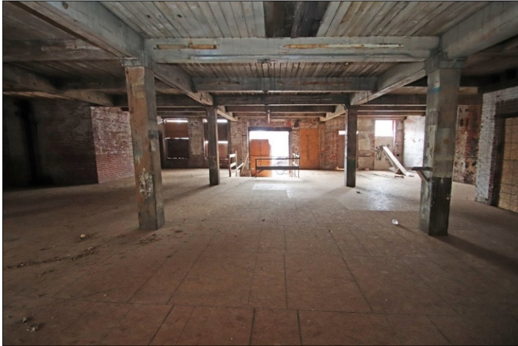
Photo 3: First floor, looking east toward the main entrance on 6 th Street.
