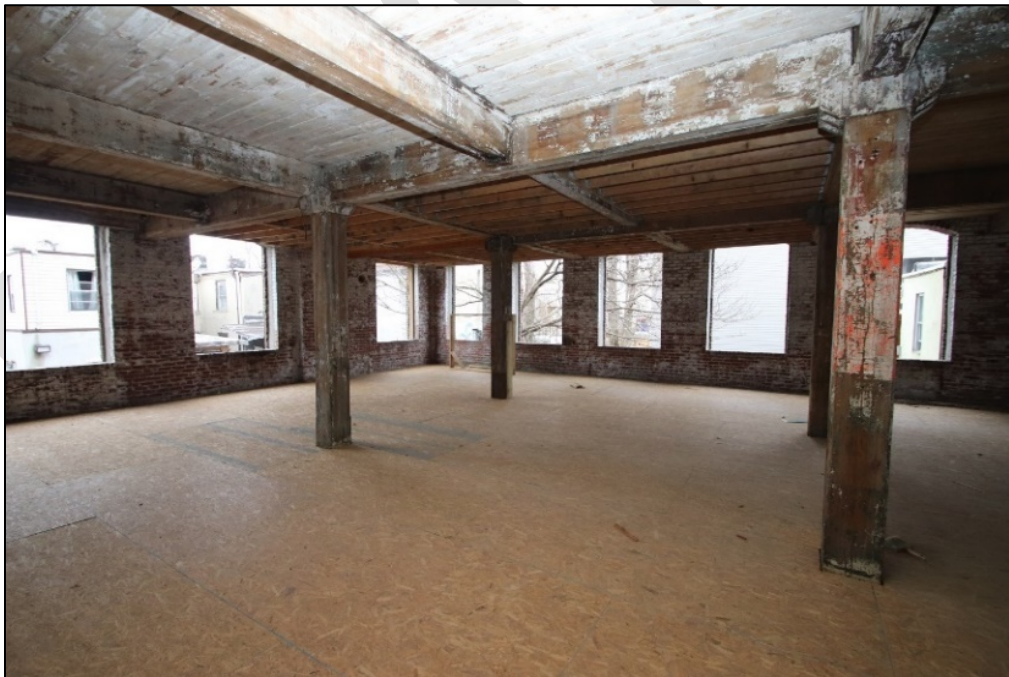
Photo 4: Second floor, looking northwest.
