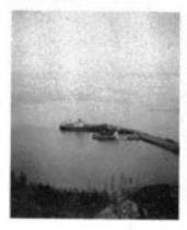
Baie Comeau was at that time only accessible by sea or by seaplane. The landing area for the seaplanes was on a lake to the North of the township. The harbour consisted of a single mole, shaped to create a basin with berthing facilities on both sides but no cranes.
