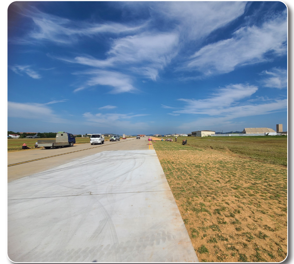
Repair Taxiway “F”
