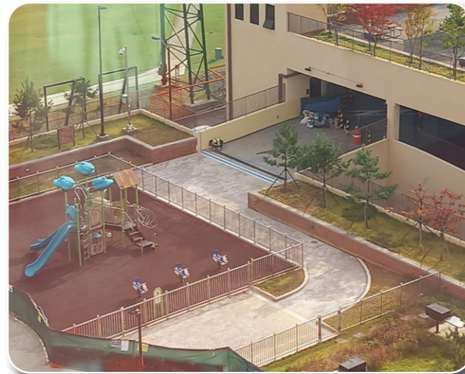
Additional Amenities and Bridge Between Towers 1& 2
