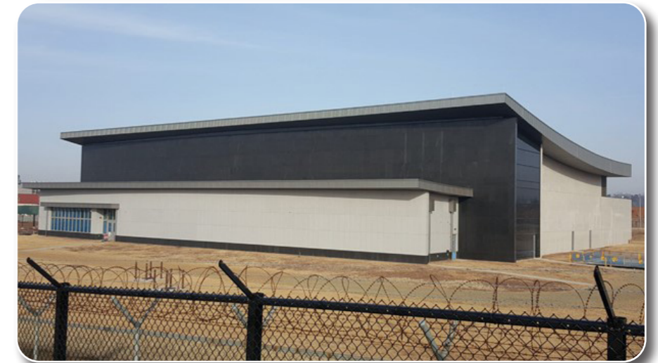
C4I030 Phase III Facility
