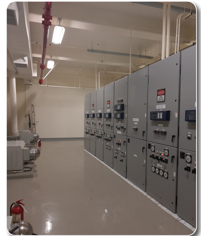
Upgrade Electrical System, Camp Henry
