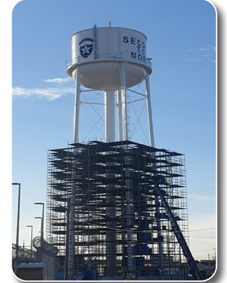
Paint 7 Water Towers
