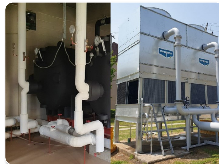
Replace Water Storage Tanks, Suwon Air Base
