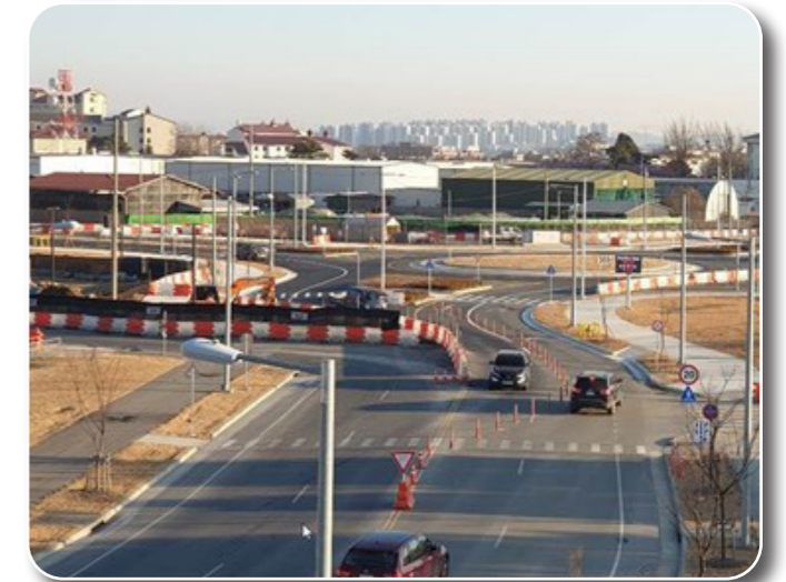
Design-Build Repair Traffic Intersection at Pacific Victors Avenue and Martin Street
