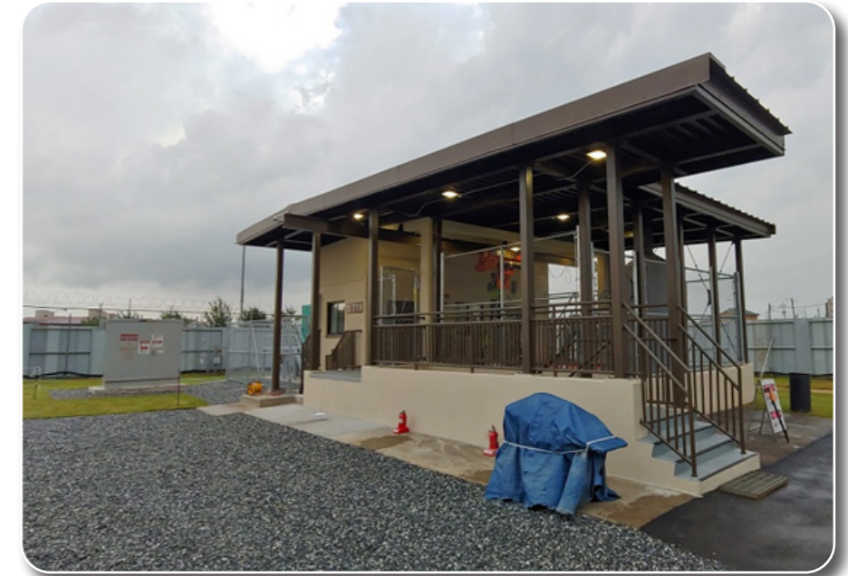
Lift Station Upgrades, S-719
