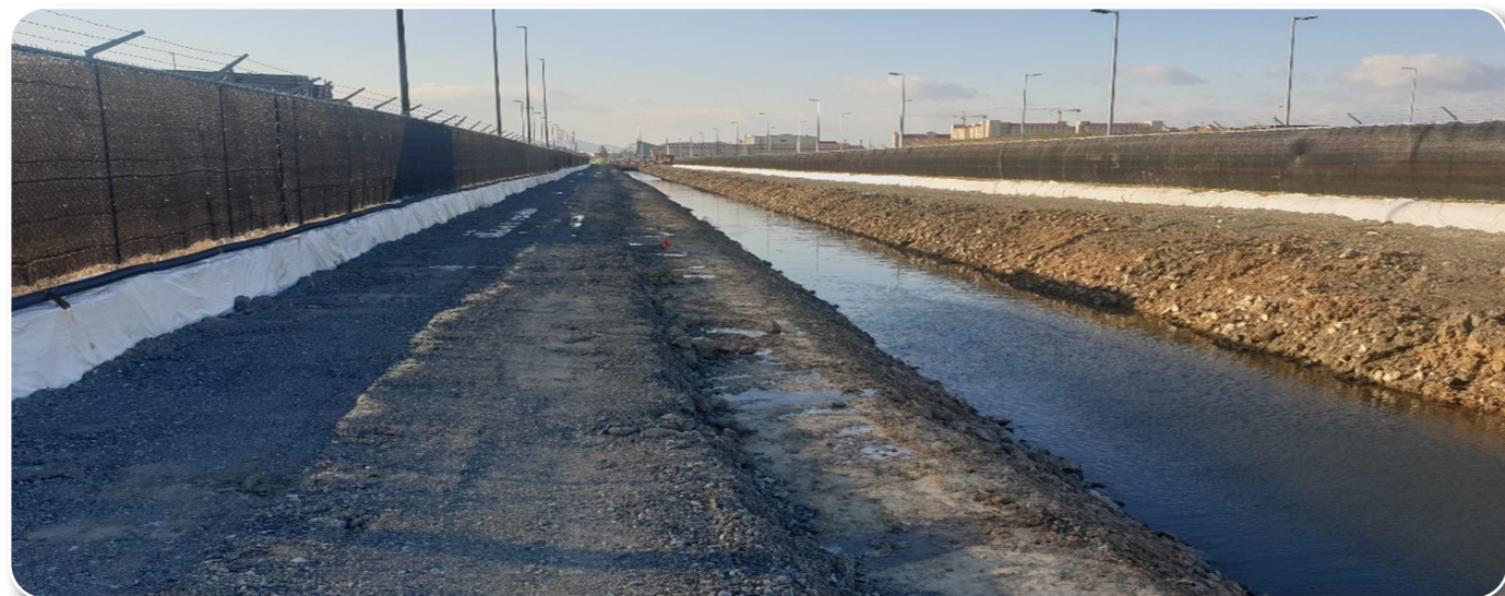
Repair Drainage Canal from 7th to 11th Street
