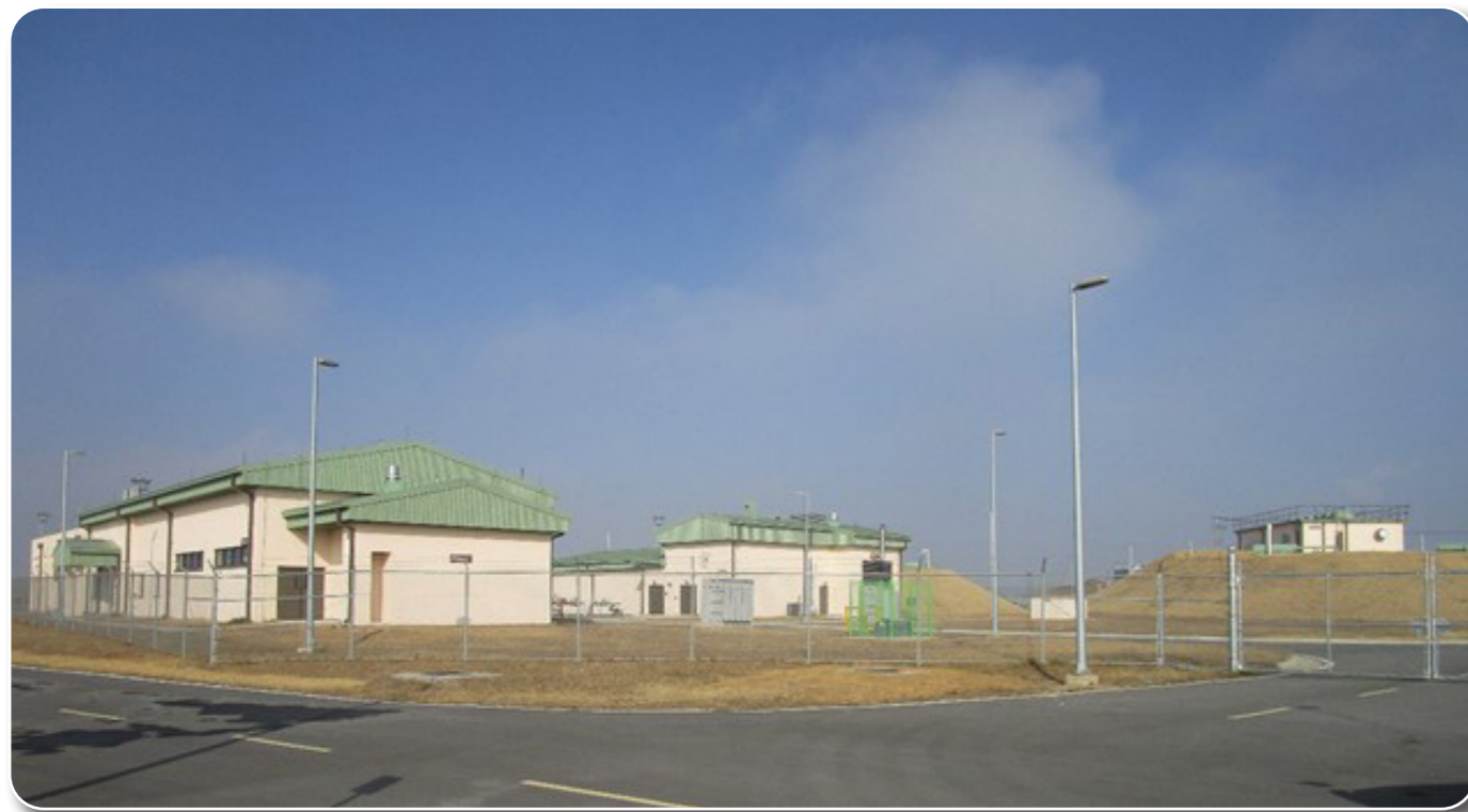
OS030 and OS031 Fuel Oil Facility
