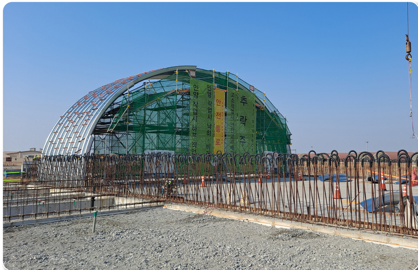
Hardened Aircraft Shelters (HAS), Phase 4-6
