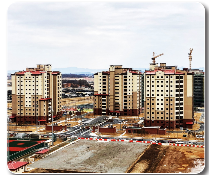
AFH100 MILCON, Family Housing New Construction
