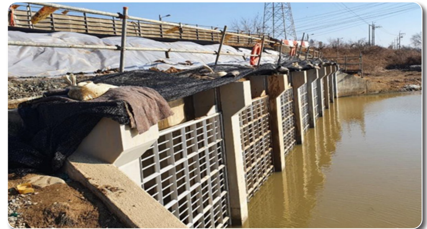
Repair Flood Gates
