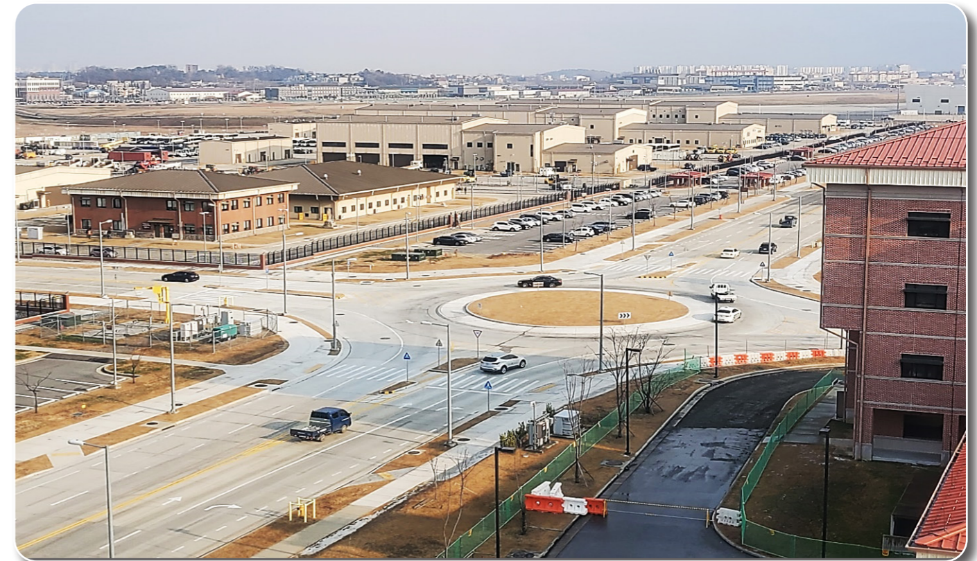
Design-Build Repair Traffic Intersection at 11th Street and Indian Head Avenue
