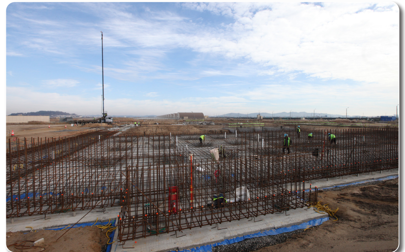
Hardened Aircraft Shelters (HAS), Phase 4-6
