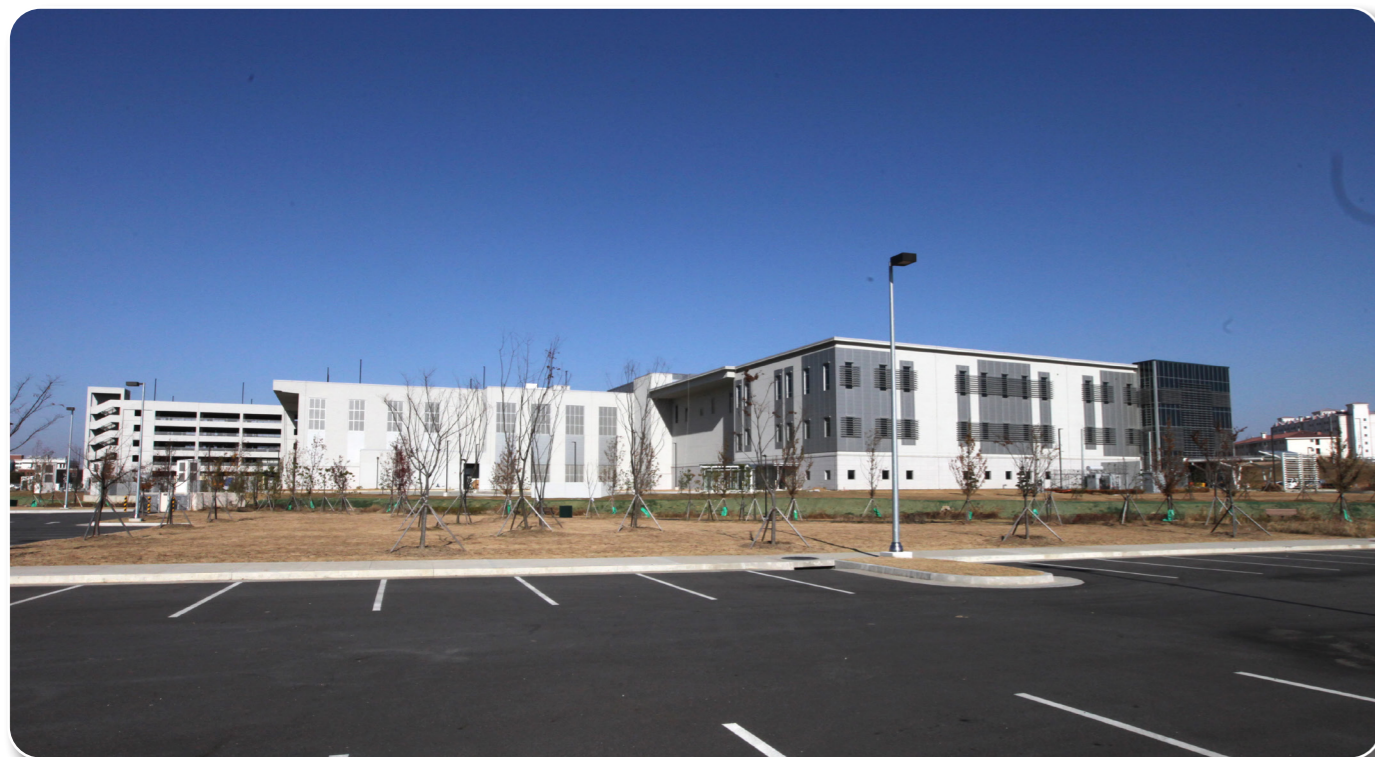
C4I010 Communications Center
