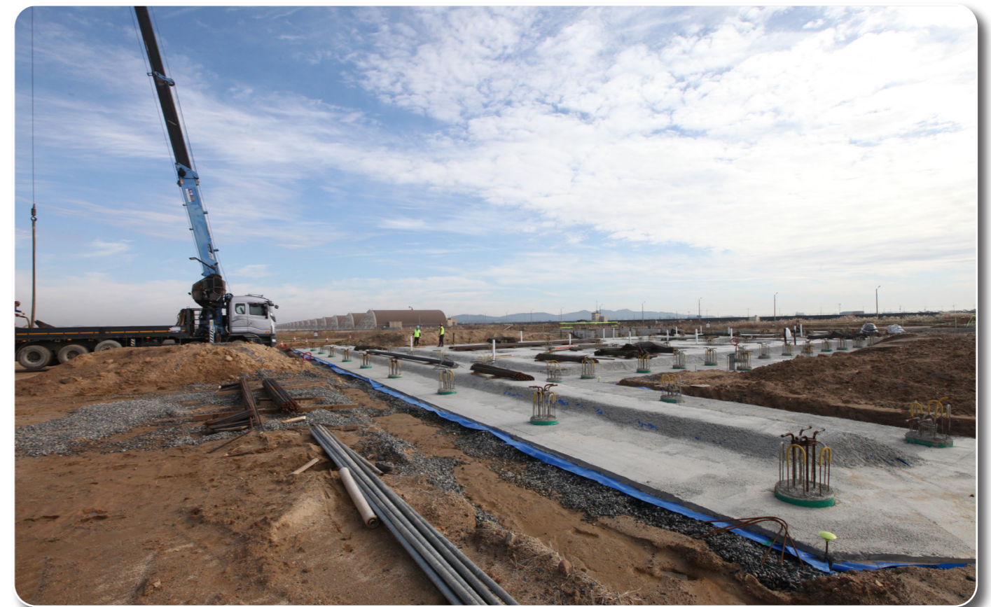
Hardened Aircraft Shelters (HAS), Phase 4-6
