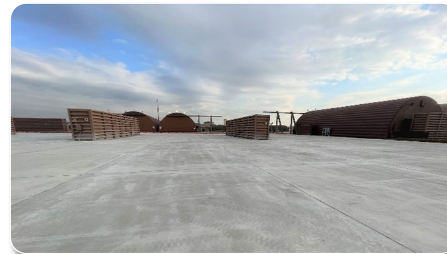
Repair Airfield Pavement, Osan Air Base
