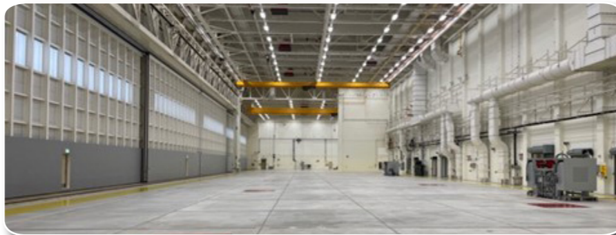
AV051 3rd MI Aircraft Maintenance Hangar Complex
