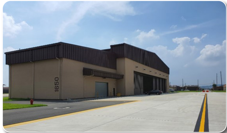
Aircraft Fuel System Maintenance Dock Exterior
