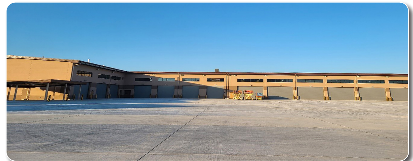
Air Freight Terminal Vehicle Maintenance Facility
