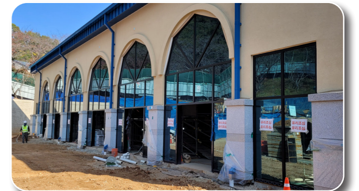
Exterior of Indoor Training Pool
