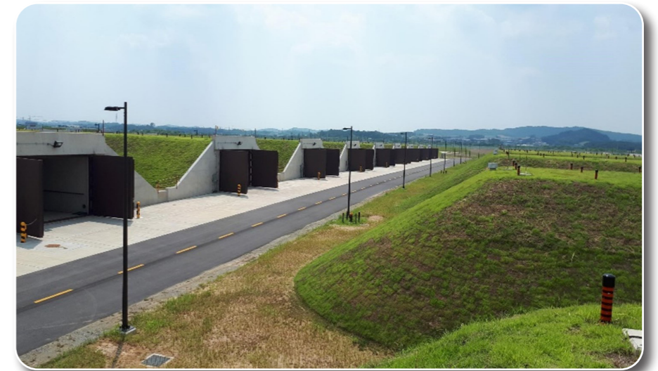
Large Munition Storage Magazines Facilities
