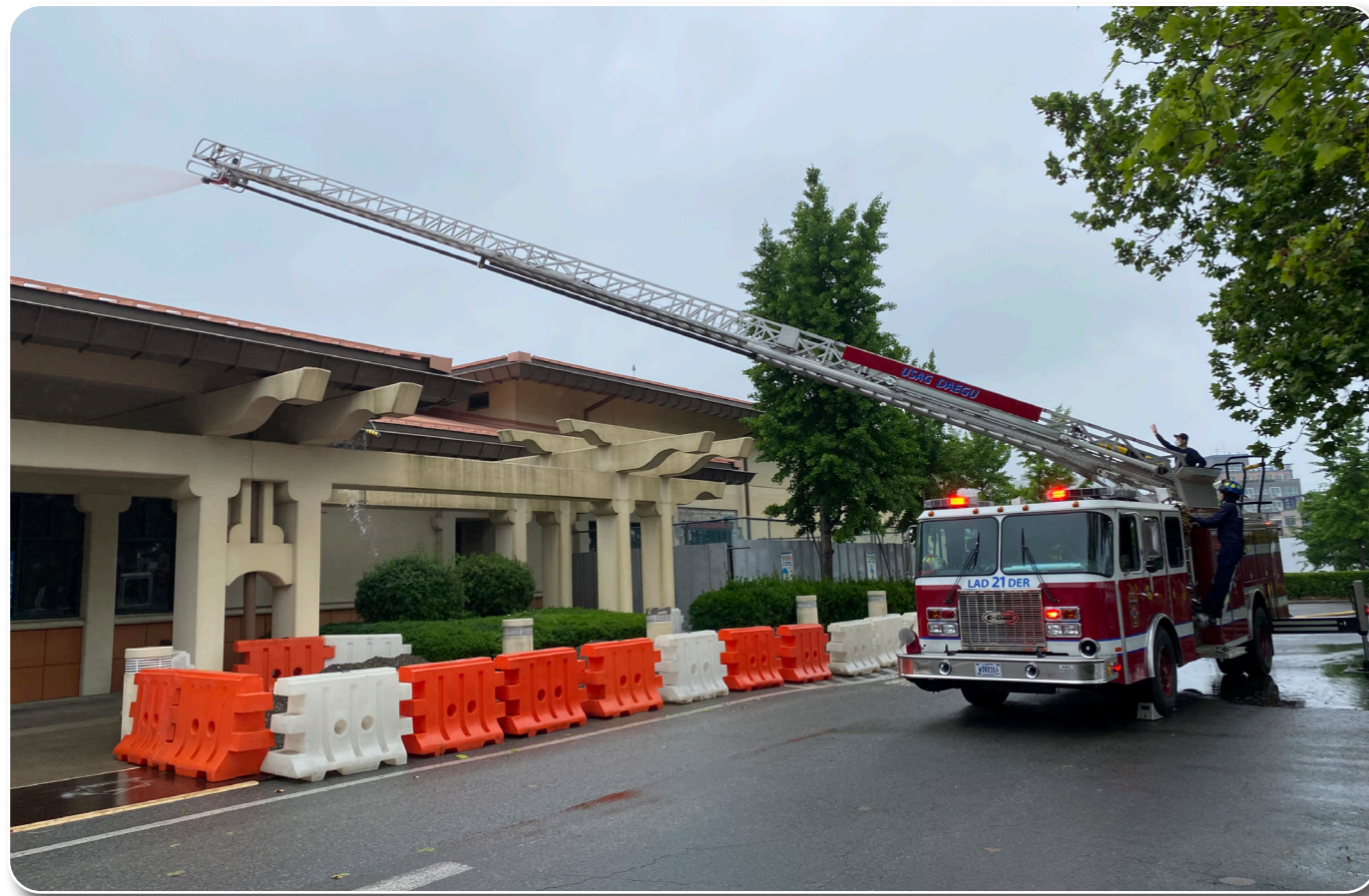
Commissary Roof Replacement, Camp Walker
