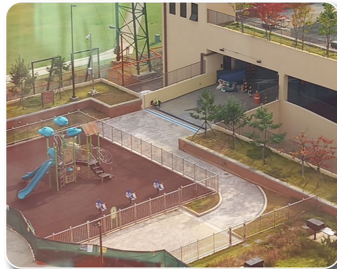
Additional Amenities and Bridge Between Towers 1& 2
