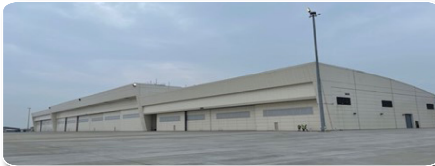
AV051 RC-7 Storage Bay, Maintenance Bay and RC-12 Storage Bay
