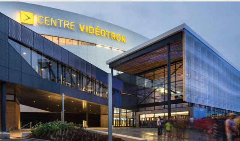
▲ Vidéotron Centre, Québec, QC LoE 366 Insulating Glass Units with Digital In-Glass Printing and Laminated Glass ABCP Architectes / GLCRM Architectes / Populous in consortium Photo: Stéphane Groleau
