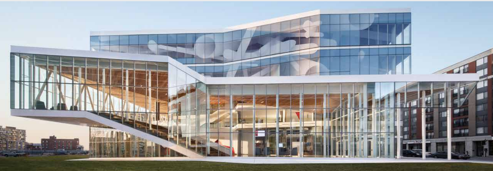
▲ École de technologie supérieure, Montréal, QC LoE 272 Insulating Glass Units with Digital In-Glass Printing MSDL Architectes
