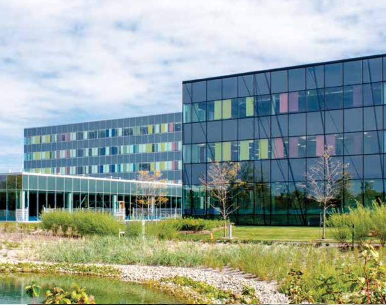
◀ Ericsson, Montréal, QC LoE 366 Insulating Glass Units with Low Maintenance Option and Digital In-Glass Printing MSDL Architectes
