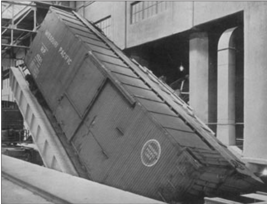
Unloading 1,500 bushels of wheat from a box car only took five to seven minutes and the service of two men at a major co-op terminal in the early 1930s, thanks to up-to-date unloading equipment.
