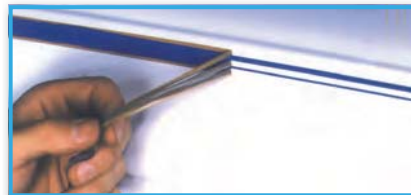
Peel off the stencil.
