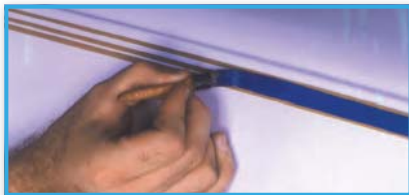
Paint over the stencil.
