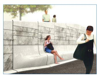
An example of a seat wall that is integrated in a retaining wall.
