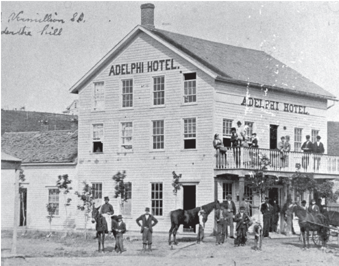
The Adelphi Hotel became a focus for firefighting efforts during the 1875 conflagration and suffered only partial damage.
