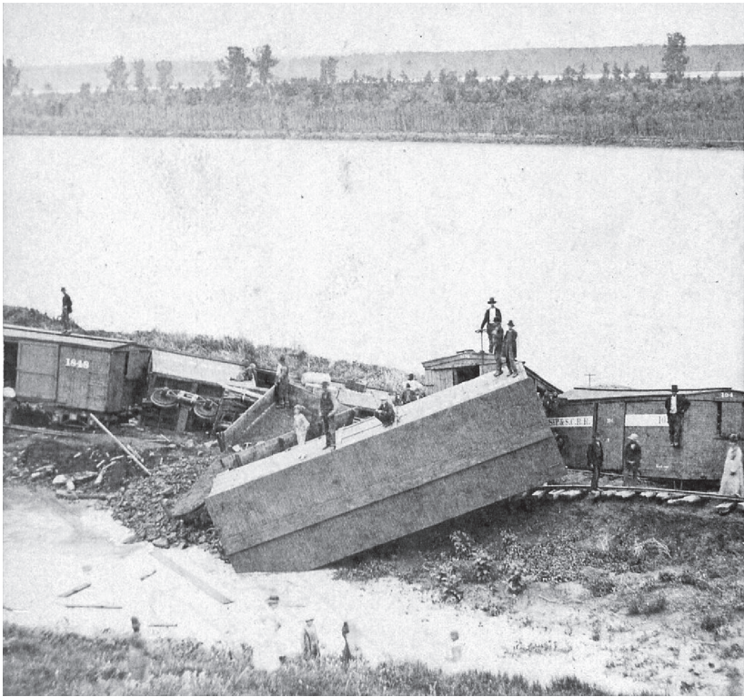
The action of the whirlpool near Vermillion was frequently a nuisance and occasionally a danger. Sometime before the 1881 flood, erosion or slumping near the whirlpool caused this train wreck.
