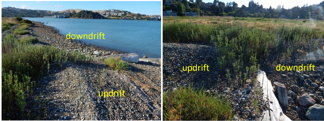
Figure 20. Log and boulder groins at Aramburu Island in June 2019, eight years after installation, are partially masked by perennial backshore vegetation (pickleweed, wester ragweed, jaumea) and gravel accumulated on the updrift side. Wood stake braces and boulders are exposed on the downdrift side.
