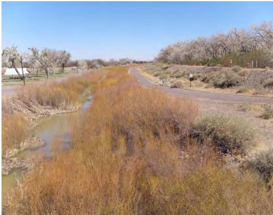
Figure 6.3 Low-Flow Conveyance Channel, Gravel Maintenance Road, and Existing Spoil Bank Looking North From the Escondida Bridge Over the Rio Grande.
