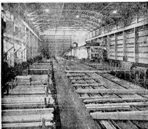
Interior Outgoing side of planing mill, 80'x560', houses the finish sorting chain. In distance at right is elevated unit conveyor leading to shipping shed.
