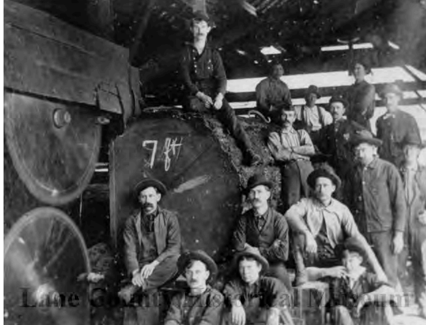
Figure 26. View of “over-and-under” or double circular saws in Booth Kelly sawmill building, c. 1900. Plant was located either at Wendling or Prune Hill. Courtesy Lane County Historical Museum, #HR23.
