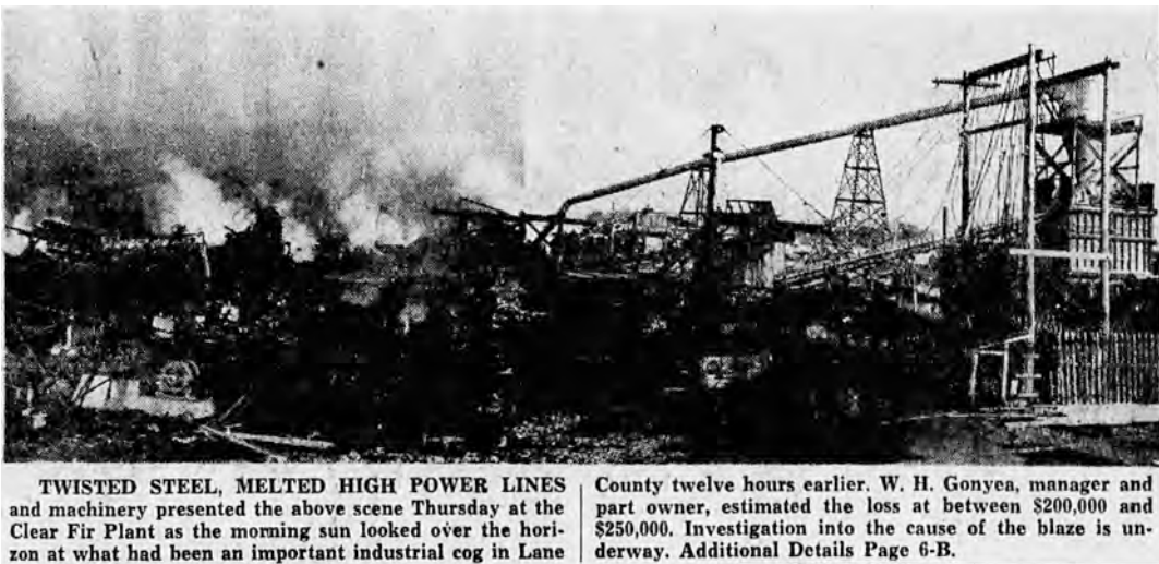
Front page photo of Clear Fir Products plant destroyed by fire (ERG 7/28/1949).
