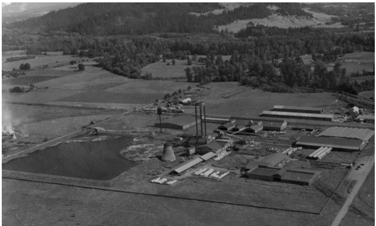
Figure 44. 1942 view of Rosboro mill. “Scene shows plant from the air; log pond, wigwam burner and water tower are at lower center, left. Main office was at 506½ Main Street, Springfield.” Courtesy Lane County Historical Museum, GN7553.
