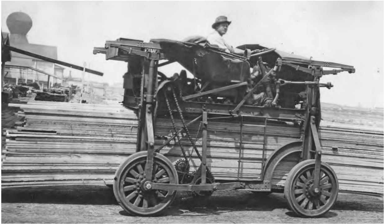
Figure 36. Booth-Kelly gas-powered lumber carrier, 1922. Courtesy Oregon State University Flickr/Frodsham photo.
