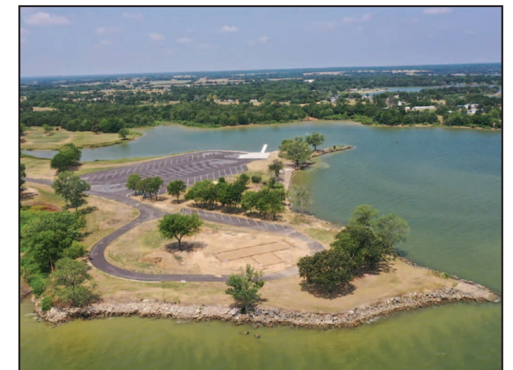
Holiday Park Construction
