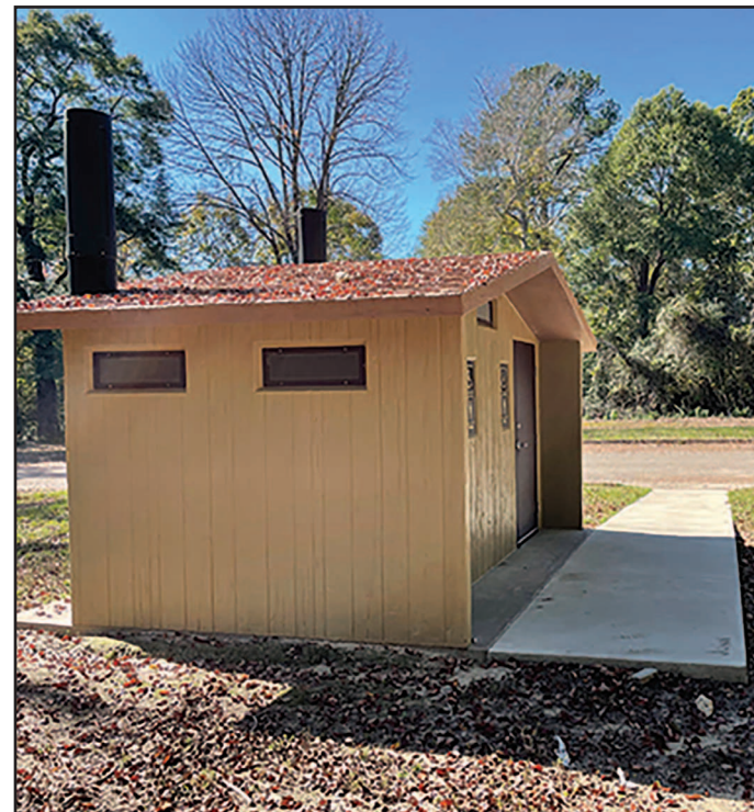
New Concrete Sidewalks at Vault Restrooms
