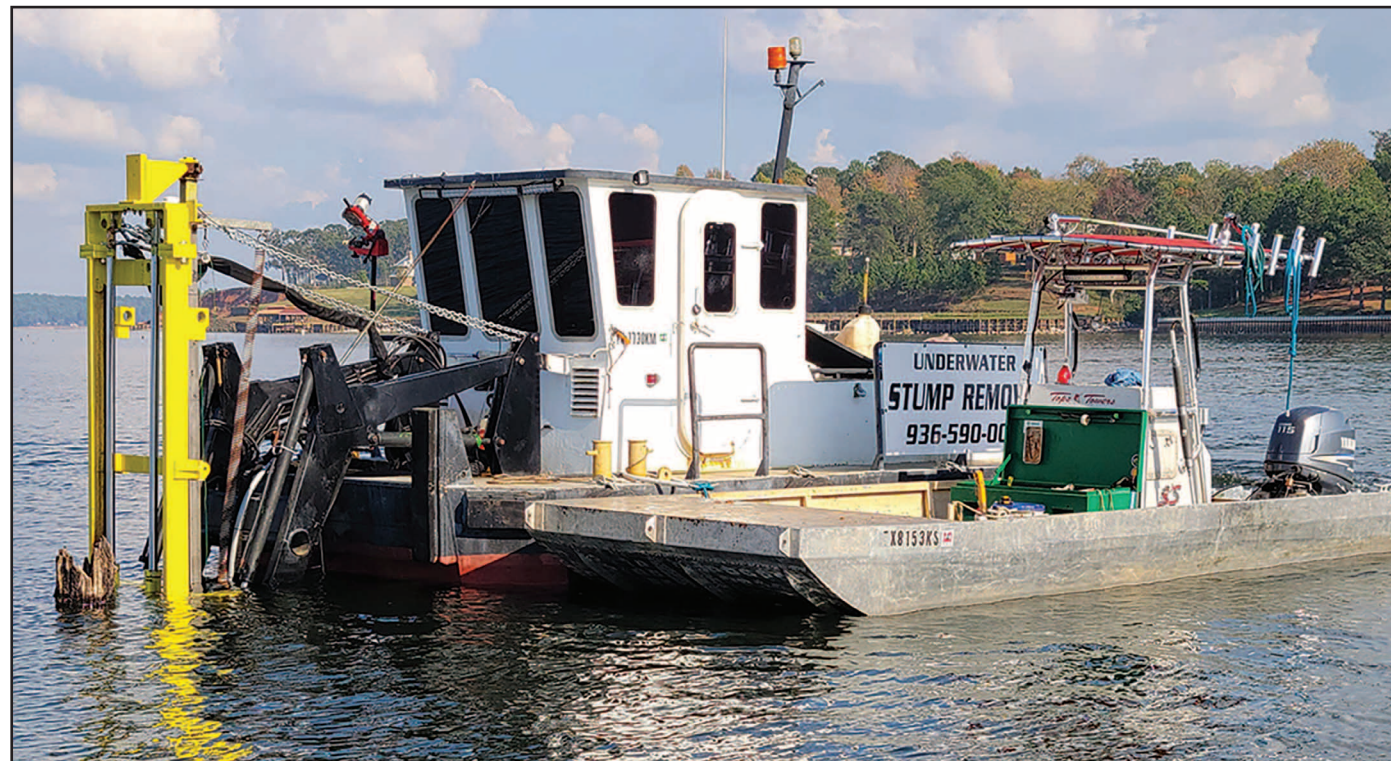
Stump Cutting for Boat Lane Improvements
