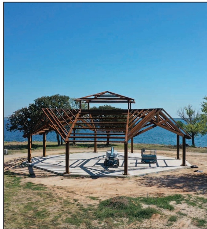
Pavilion Construction at Lake Tawakoni Recreation Site
