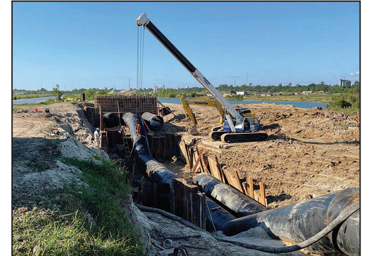
Womack Siphon Construction
