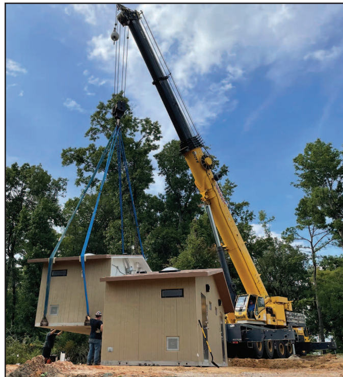
New Restroom Facility at Ragtown
