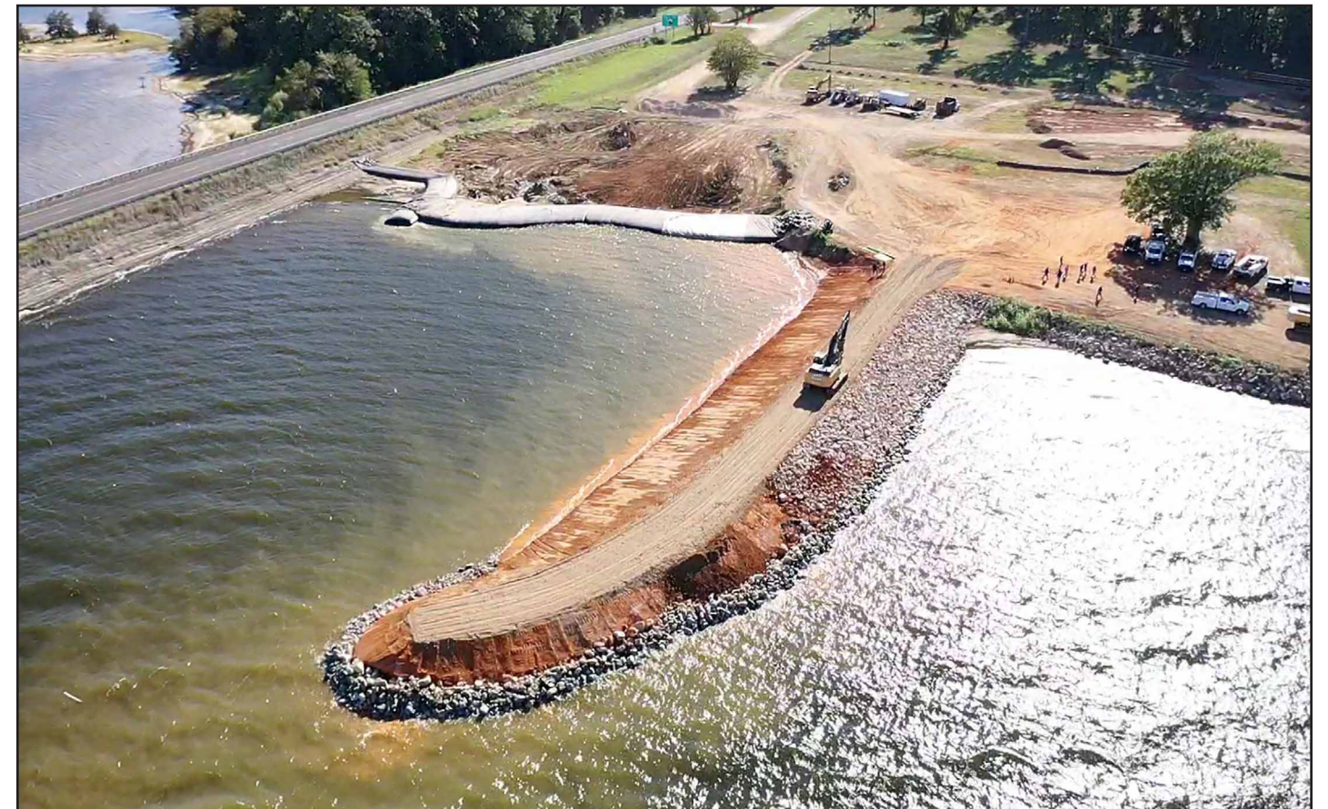
Construction at Pendleton Park
