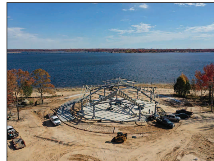
Pavilion Construction at Caney Point
