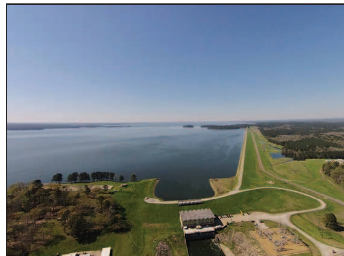
Toledo Bend Dam and Reservoir
