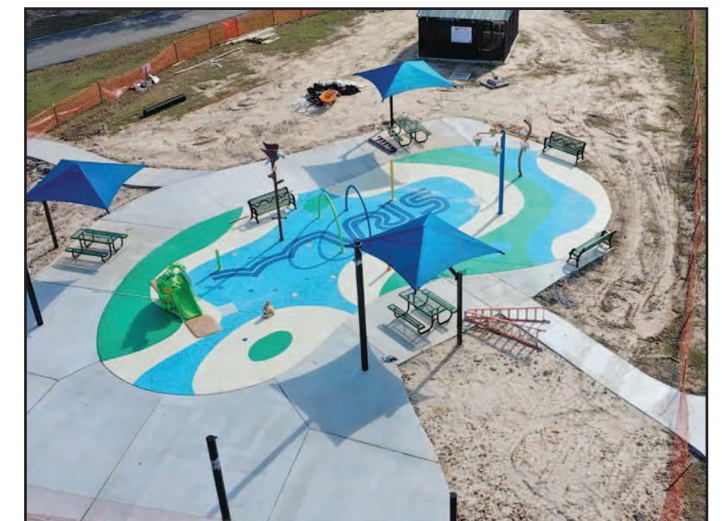
Splash Pad Construction at Swearingen Park
