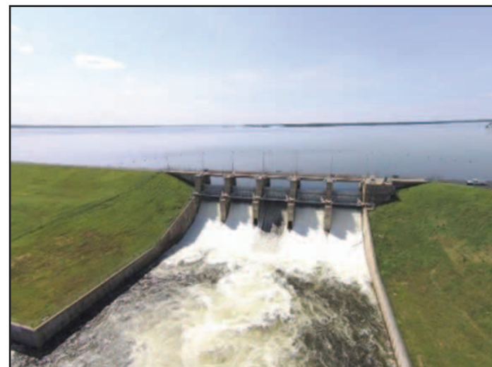
Lake Fork Dam and Reservoir
