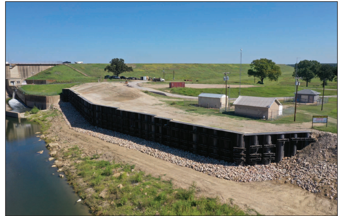
Completed Spillway Channel Bank Stabilization Project
