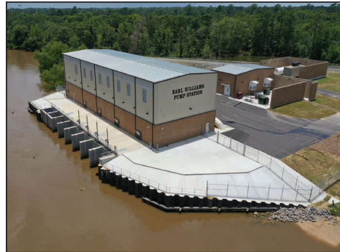
Earl Williams Pump Station
