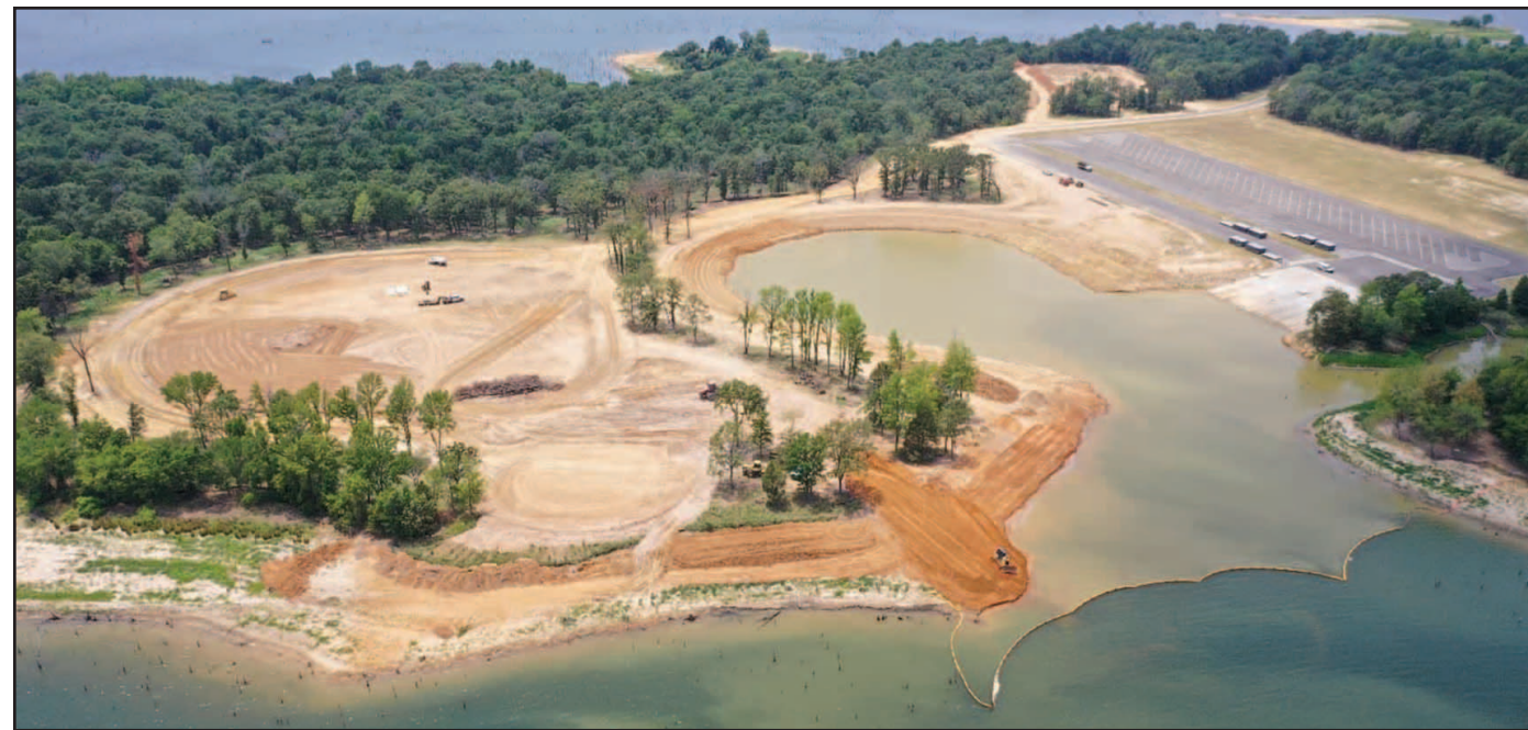
Construction at Caney Point Recreation Area
