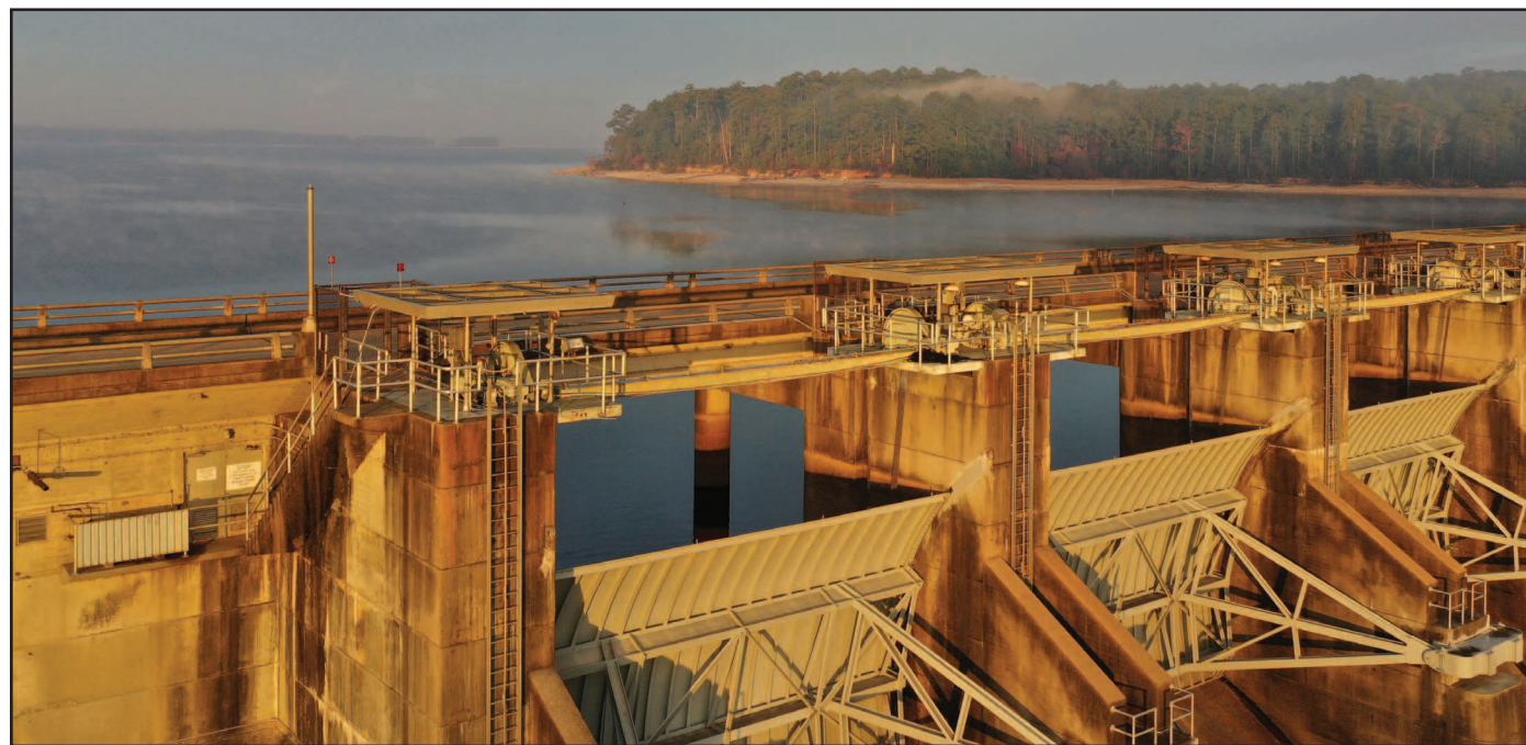
Toledo Bend Spillway Gates
