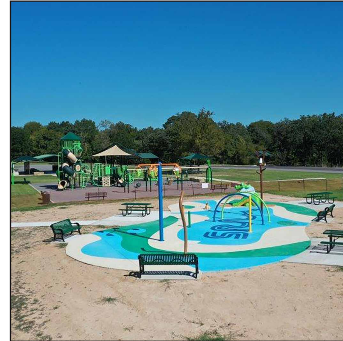
Construction of Splash Pad at Swearingen Park
