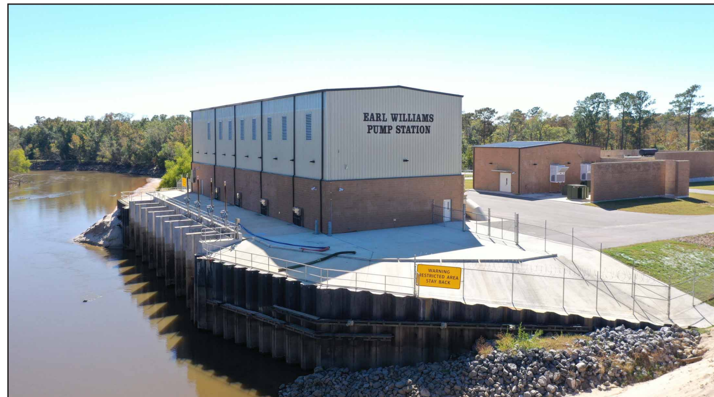
Earl Williams Pump Station
