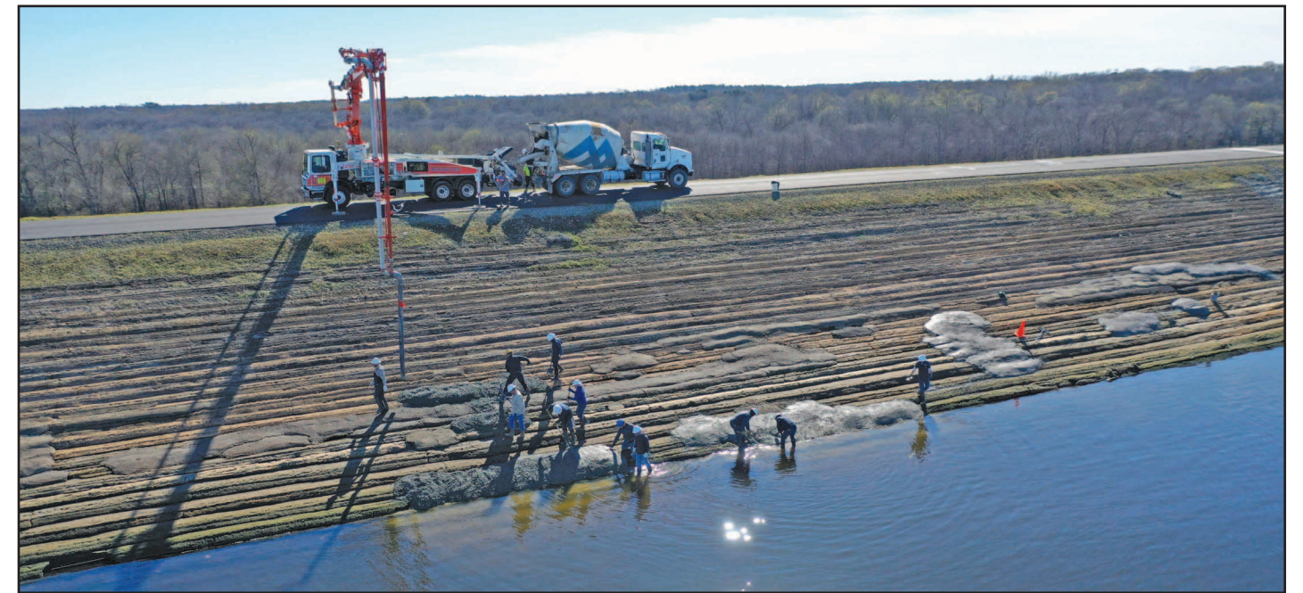
Soil Cement Repairs on the Dam Face
