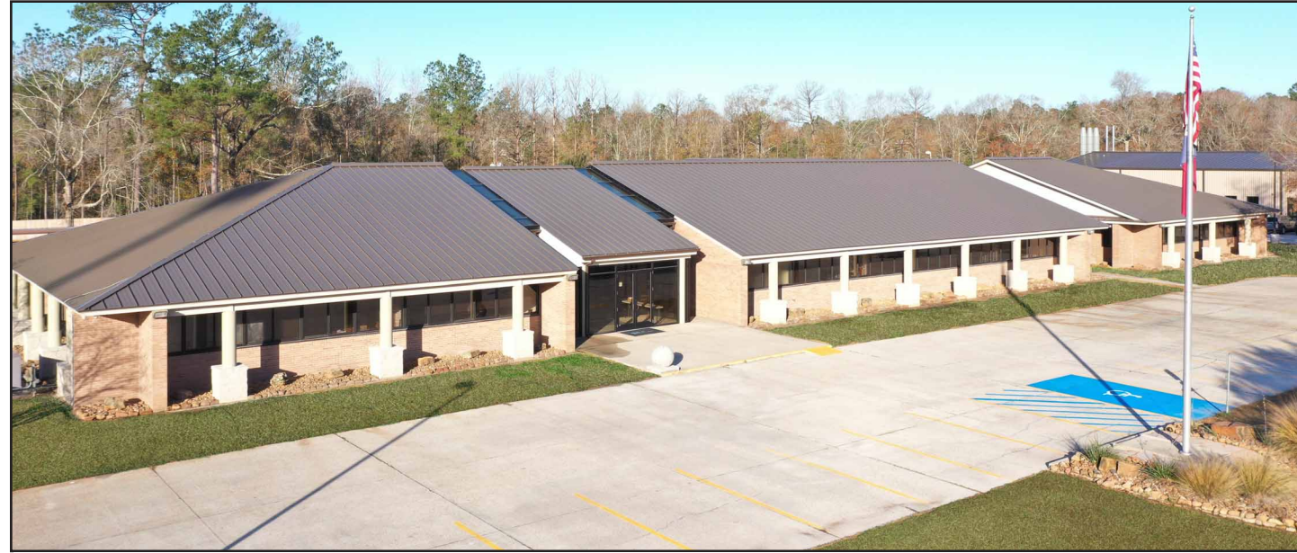
Sabine River Authority General Office
